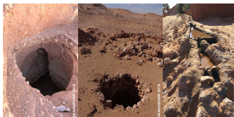
Fig. 3. Worked stone masonry wells and Ifli in Taghamt Enoura’ and Izendha’, Taguelzi (Illili Mahrouq, 2018).
