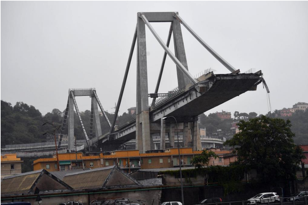
Fig. 1.2. Aftermath of Morandi Bridge collapse, Genoa, Italy (August 2018). The tragedy killed 43 people and left 600 homeless [6].
