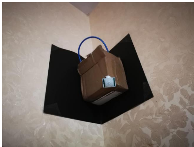
Figure 43. Implementation of the detector (installed)
