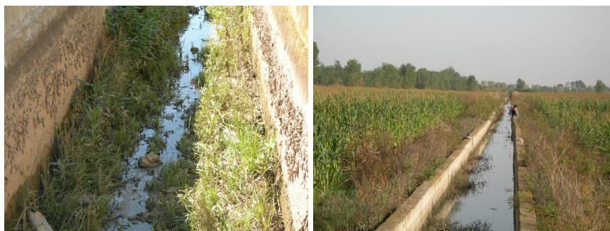
Figure 5.9: Irrigation canal used for the field experiments.
