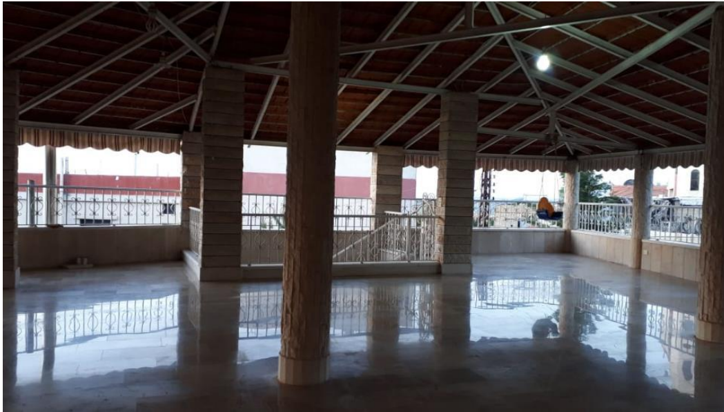
Figure 189 1st floor terrace Source: Author (2019)
