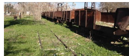
Figure 39 Abandoned train railway from Riyaaq - Bekaa source: Author (2017)
