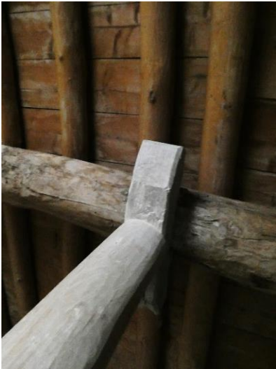
Figure 4 "Shama'a" (Column) with the "Taj" (Capital) in a dwelling in El Nabisheith Source: Author (2018)
