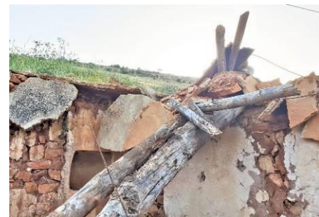
Figure 55 Fallen ceiling of an old structure, showing the material used to construct this vernacular dwelling. Source: Author (2020)
