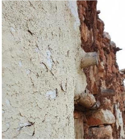
Figure 83 Exterior wall Source: Author(2020)
