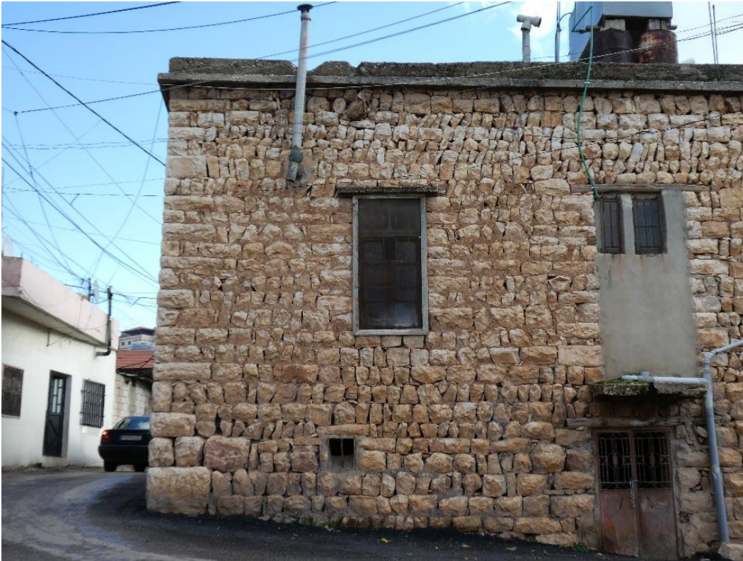
Figure 99 Dwelling P-1 Exterior Source: Author( 2018)
