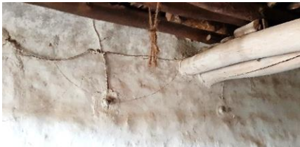
Figure 112 Light switch installation next to the wooden beam Source: Author (2018)
