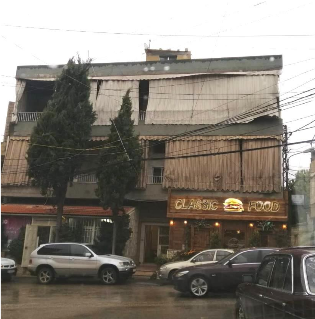
Figure 174 Frontal facade of the building Source: Rania Mohammad (2019)
