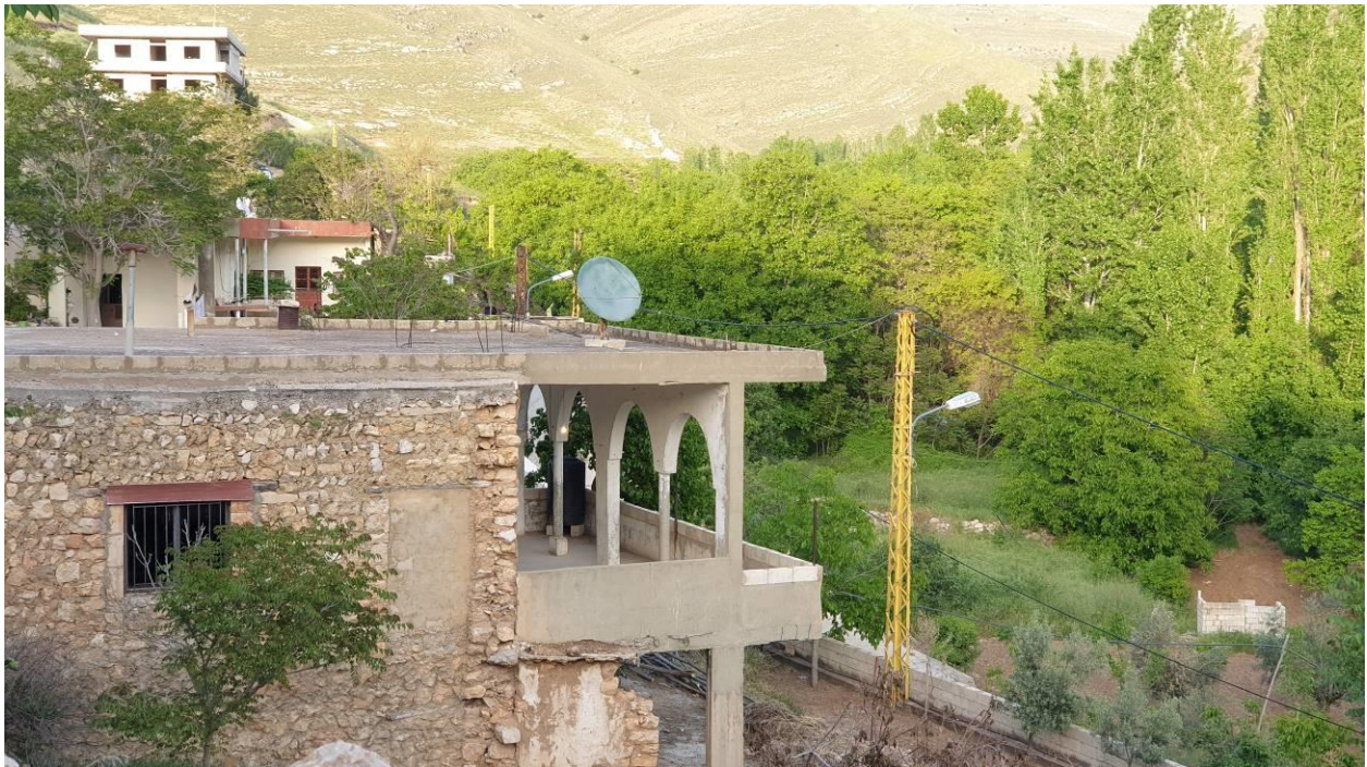
Figure 283 A modified vernacular house, where we can see how concrete arches are added against an old stone and mud house Source: Author (2020)
