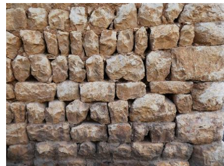
Figure 28 Stone Facade Wall Source: Author (2018)
