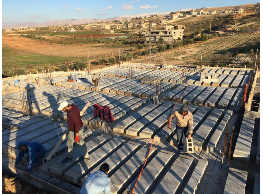
Figure 208 Preparing steel for raft foundation Source: Author (2018)
