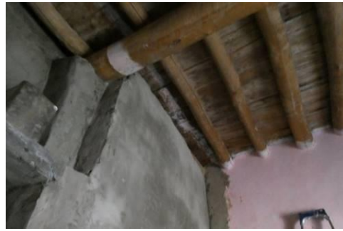
Figure 119 Interior wall plastered with a concrete base material Source: Author (2018)
