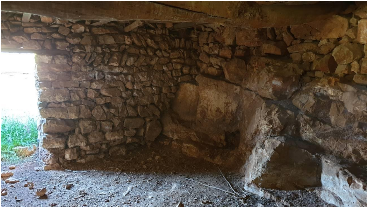
Figure 278 Interior of an old dwelling built against the natural stone of the mountain. Source: Author (2020)
