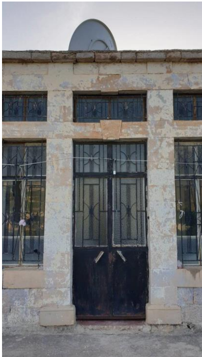
Figure 285 A vernacular dwelling with a key stone on its lintel that says built in 1947. This dwelling is the only house with ornamented façade and clearly cut stones found. Source: Author (2020)
