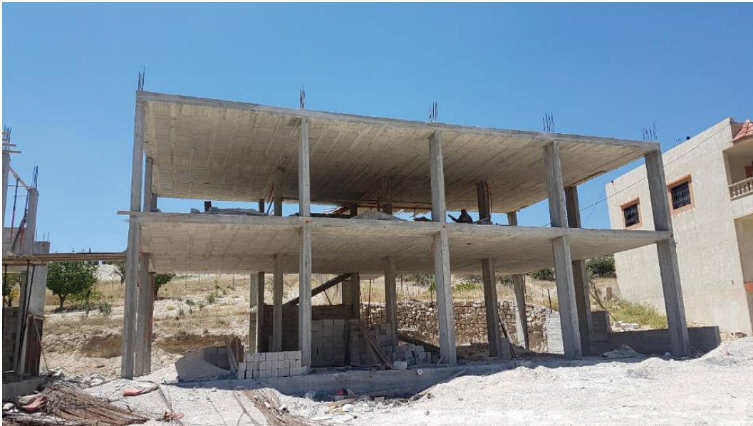
Figure 224 Construction in process. Block A source: Author (2018)
