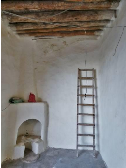
Figure 29 Image from a dwelling in the Bekaa valley Source: Author (2018)
