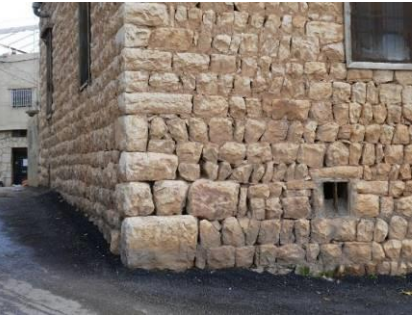
Figure 100 Dwelling P-1 Exterior Source: Author (2018)
