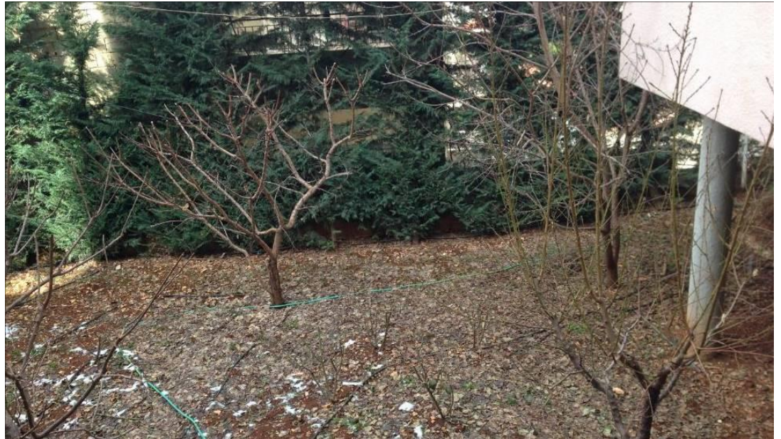
Figure 191 Photo of the garden 50 cms above the basement level. On the right we can see the new column added to create a backyard terrace. Source: Author (2018)
