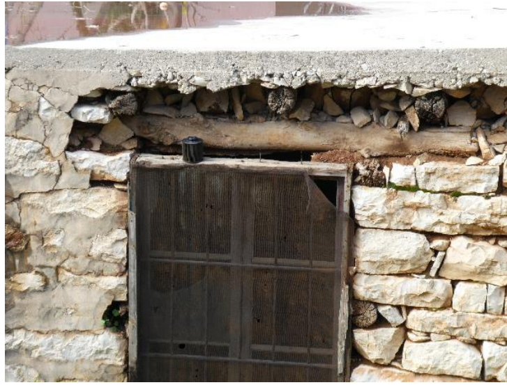
Figure 132 Mud roof topped with a concrete and pebble mix
