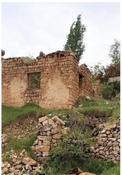
Figure 32 A vernacular dwelling in Janta - Al Nabisheith Source: Author (2020)
