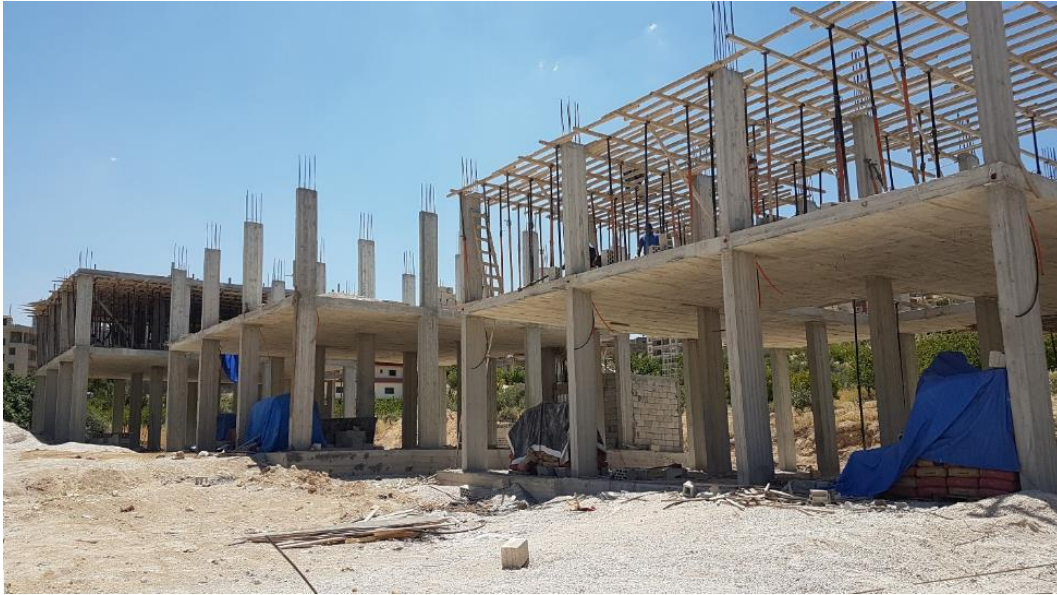
Figure 223 Construction in process. Block B, C, and D source: Author (2018)
