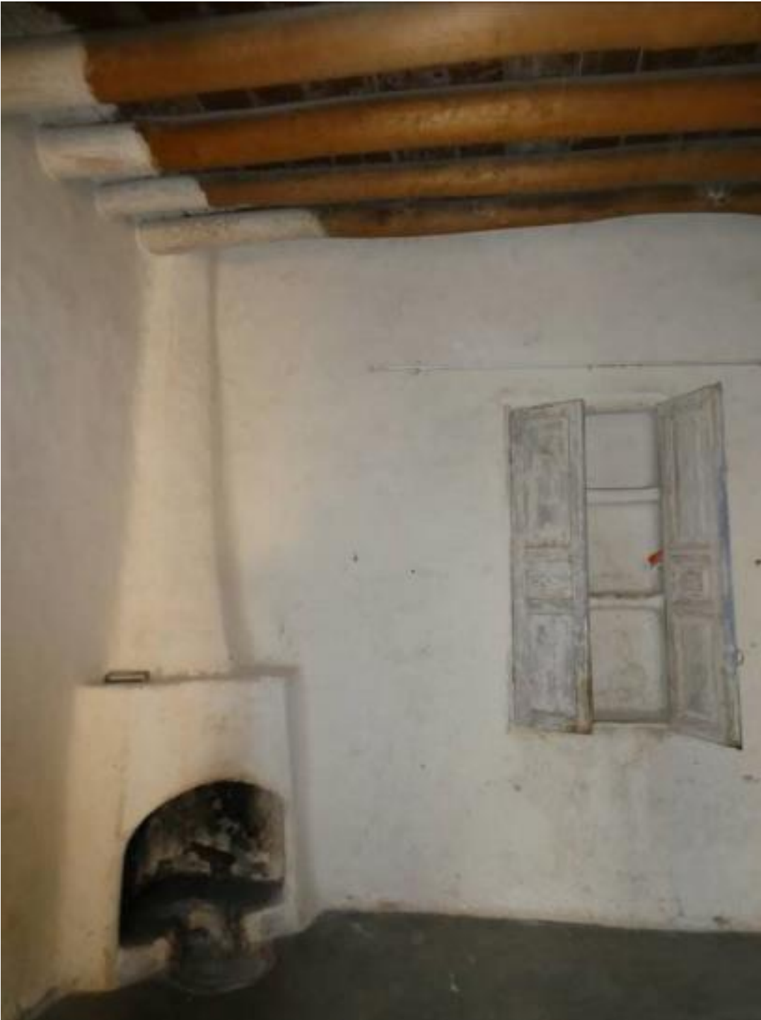
Figure 173 Chimney in the living space. Source: Author (2018)
