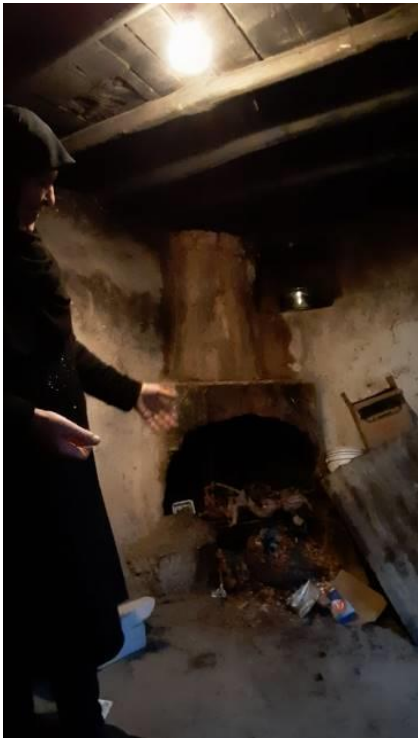
Figure 150 Image of the old chimney located in space "1". Source: Author (2018)
