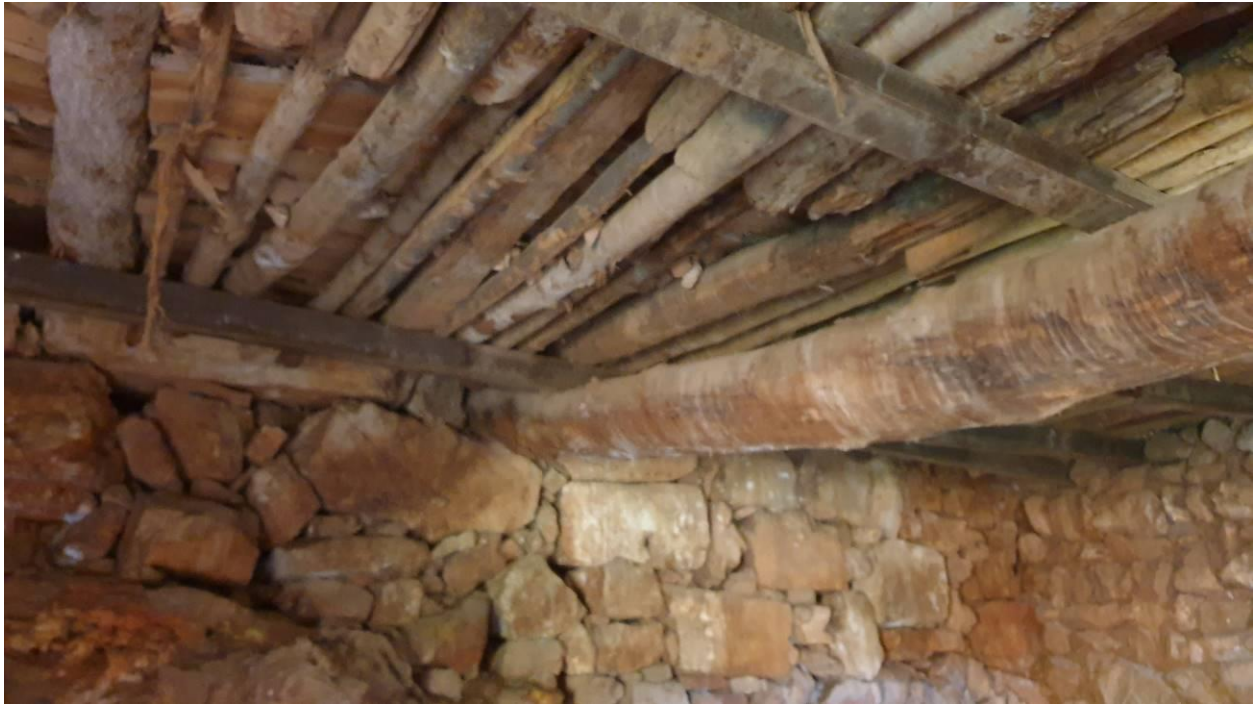
Figure 282 Interior ceiling of a vernacular dwelling Source: Author(2020)
