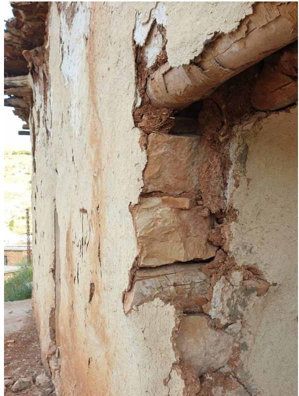
Figure 276 Wooden door lintel + wall detail Source: Author(2020)
