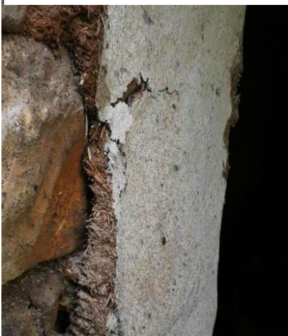
Figure 84 Detail of a mud plaster and wall construction Source: Author (2019)
