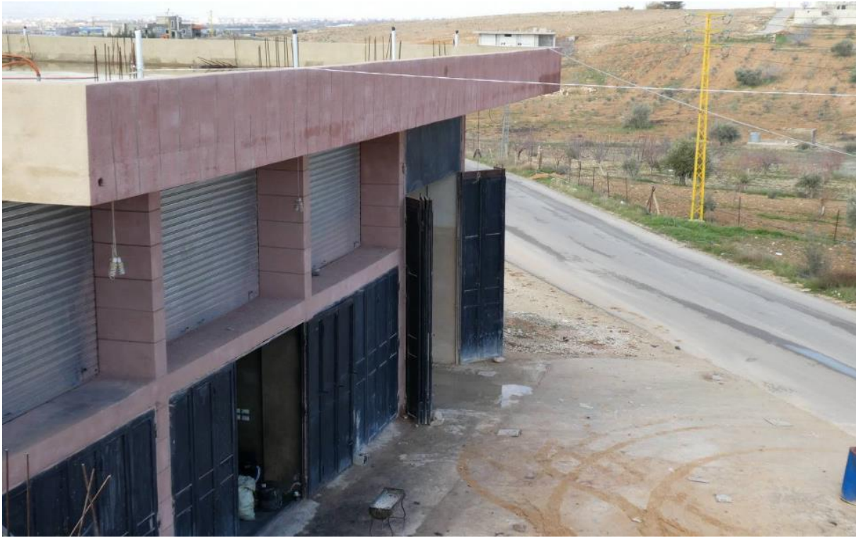
Figure 211 Ground floor raft foundation just poured Source: Akram Moussawi (2019)
