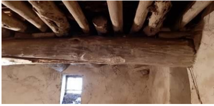
Figure 109 Primary and secondary beams Source: Author (2018)
