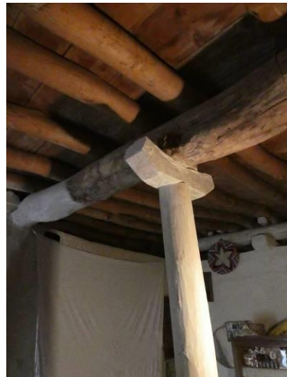
Figure 91 both images are construction samples of the detail above. Source: Author (2018)
