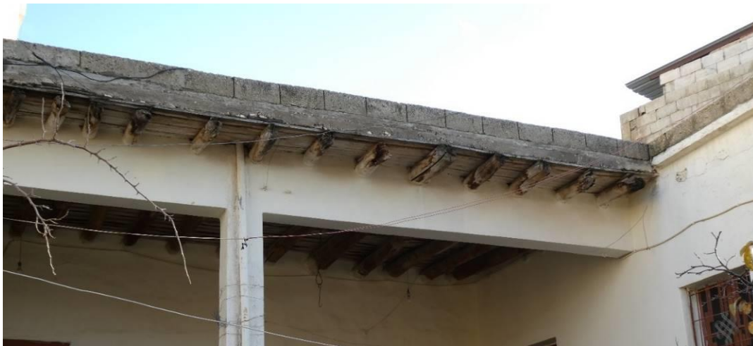
Figure 30 Adapted vernacular ceiling to new construction materials Source: Author (2018)
