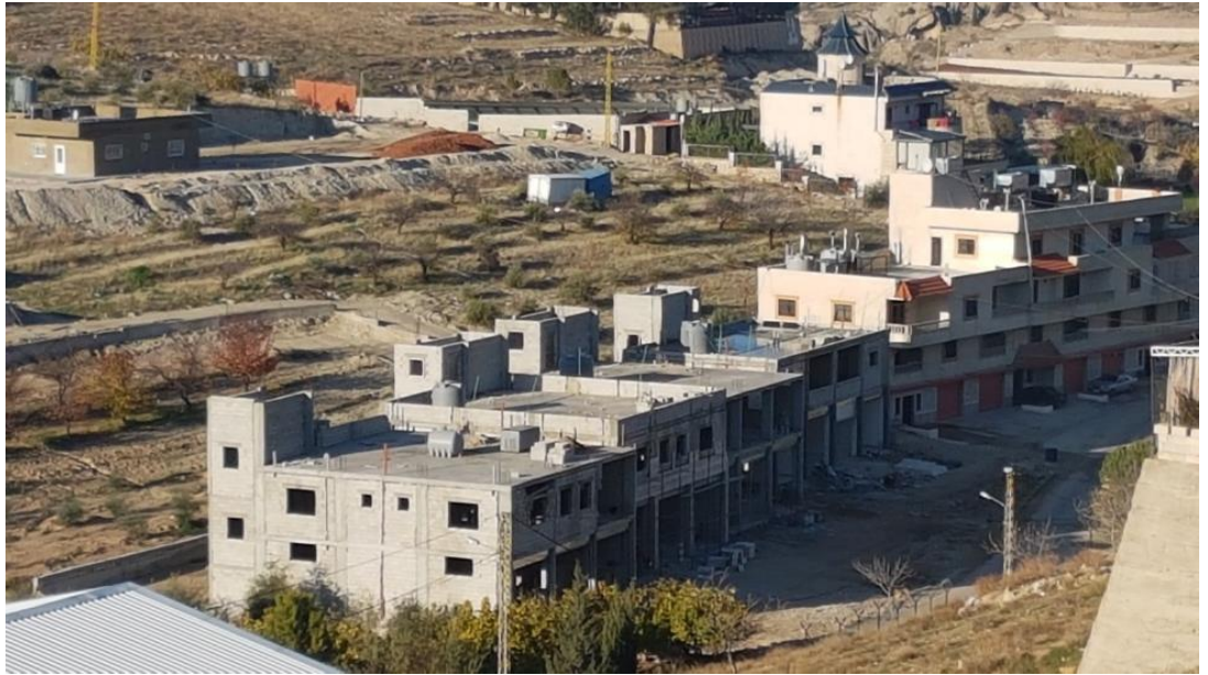
Figure 218 PP-3 Buildings facade facing the main road. Source: Author (2018)
