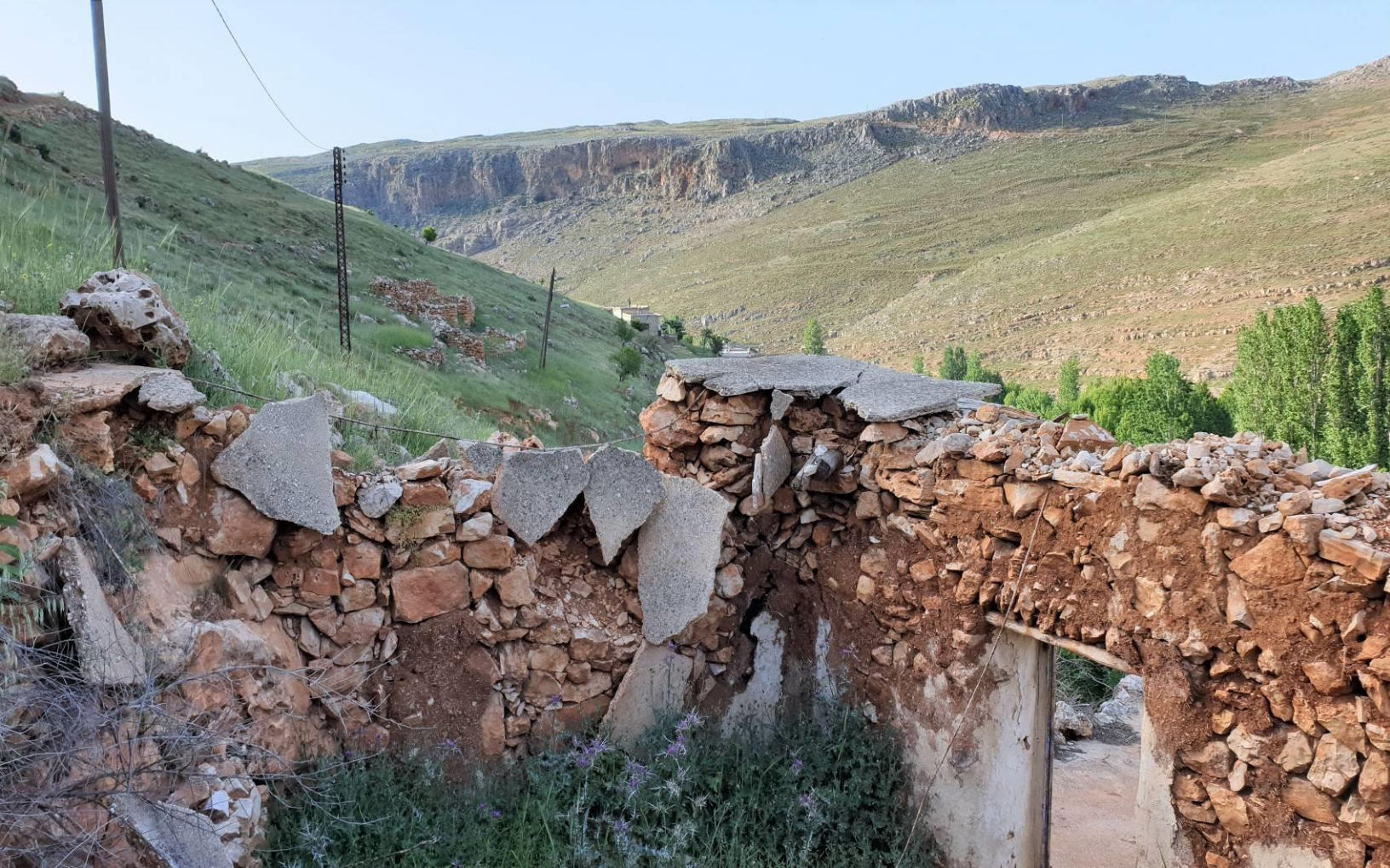
Figure 94 Vernacular dwelling emerging from the landscape overlooking the eastern mountains Source: Author (2020)
