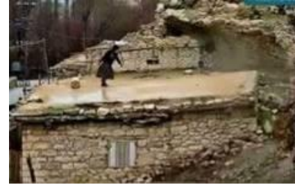
Figure 87 Image of a woman using the “Mahdale” on the ceiling by the end of summer. Source: Unknown (1950’s)
