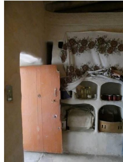
Figure 42 Interior closets made of mud to absorb humidity Source: Author (2018)
