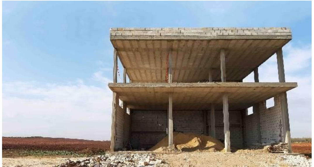
Figure 227 PP-4 Dwelling facade, picture taken from the main road. Source: Author (2018)
