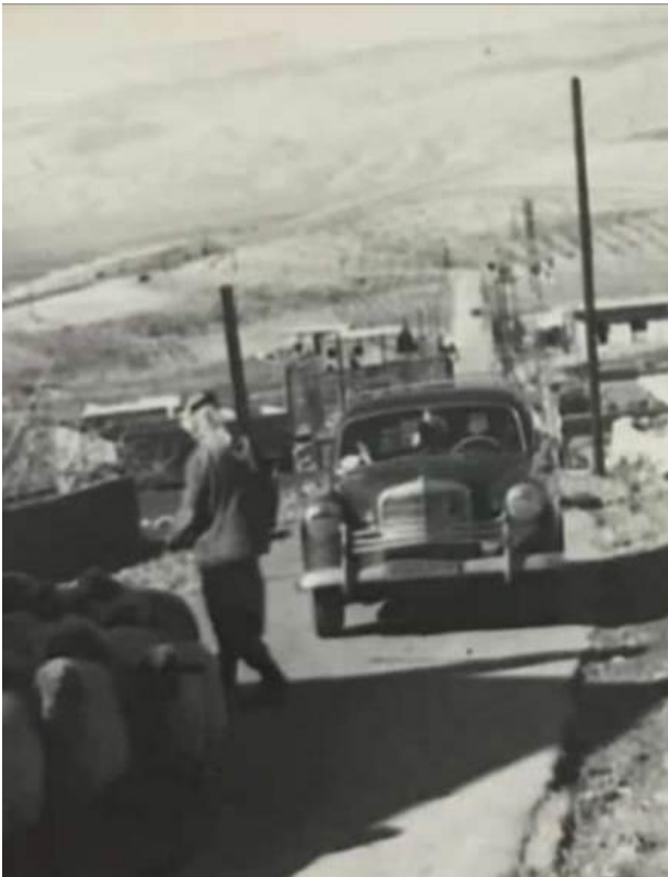
Figure 248 Nabisheith Bekaa Road Source: Unknown (1970's)
