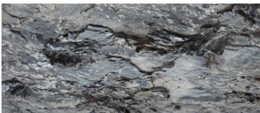
Figure 7. Delamination example from the site.
