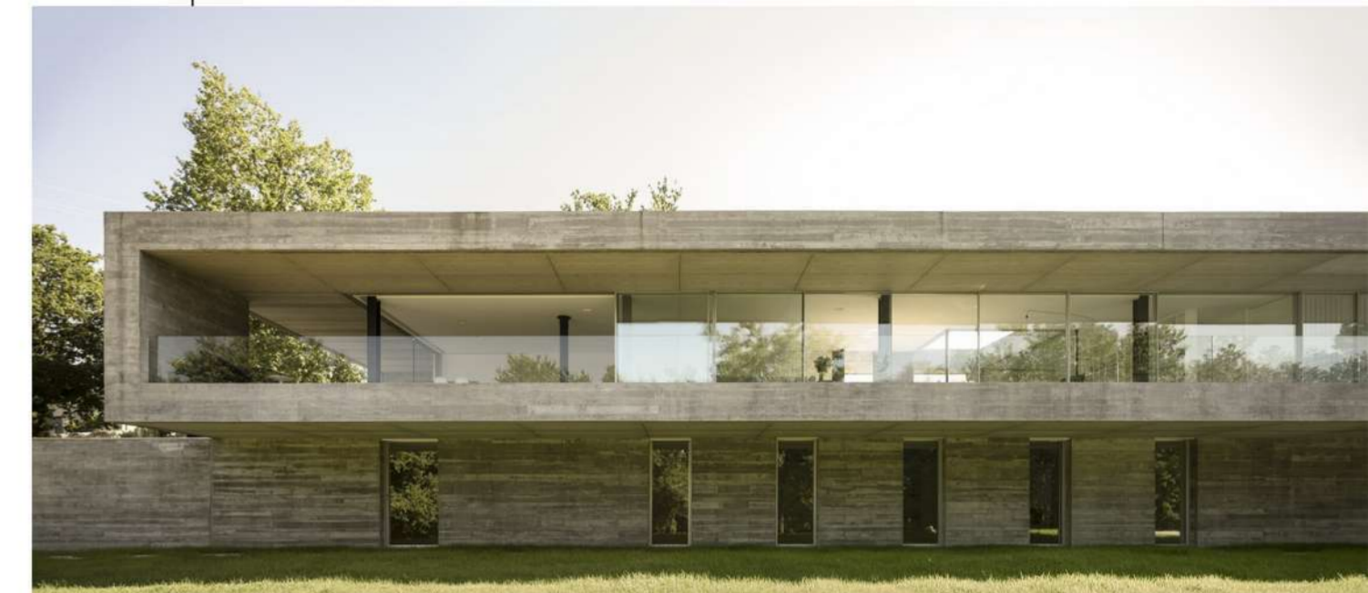
Ref: casa de sambade de Spaceworkers
