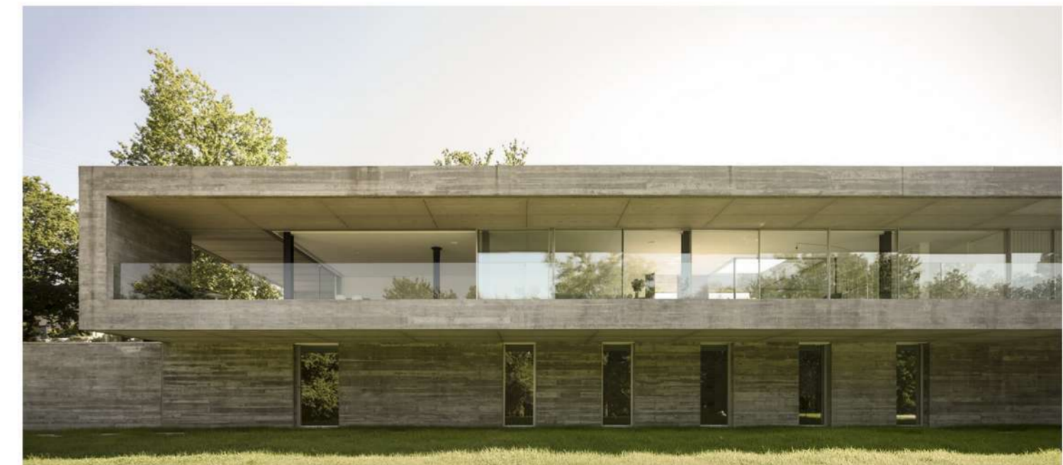
Ref: casa de sambade de Spaceworkers
