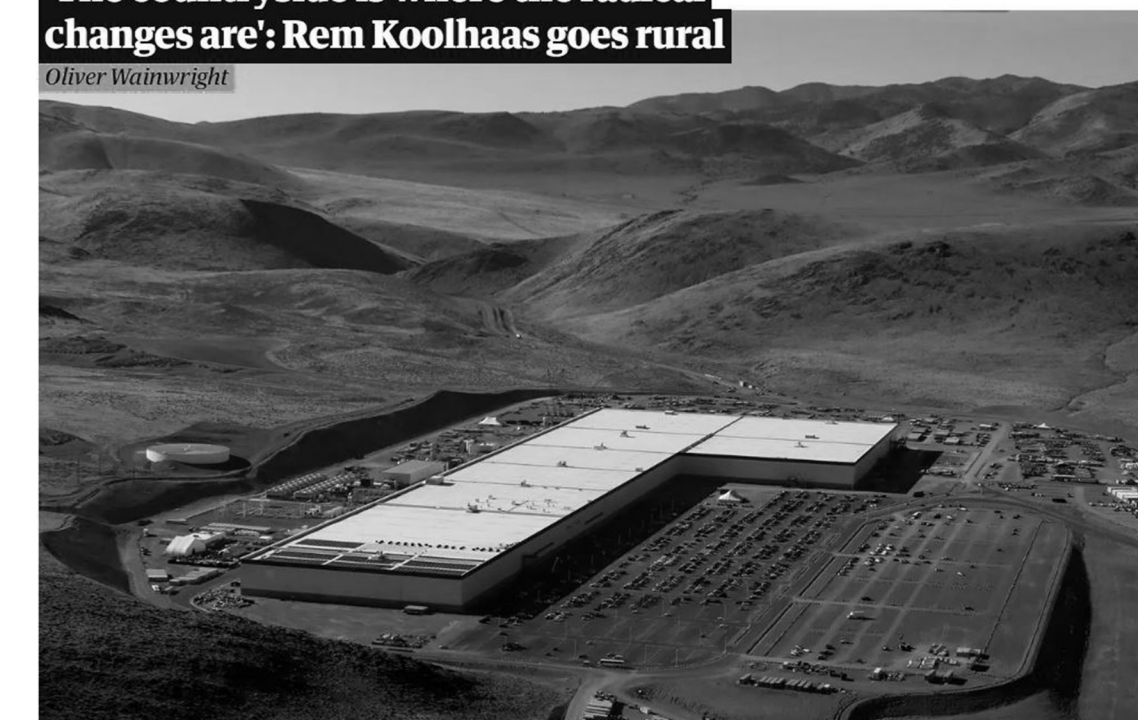
▲ 'Its boredom is hypnotic, its banality breathtaking' ... the world's largest building, the Tesla Gigafactory, embodies the new architecture. Photograph: Bob Strong/Reuters
