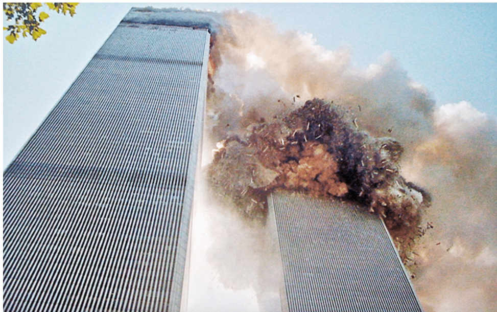
Figure 1.3: Collapse of the World Trade Center. From [5].
