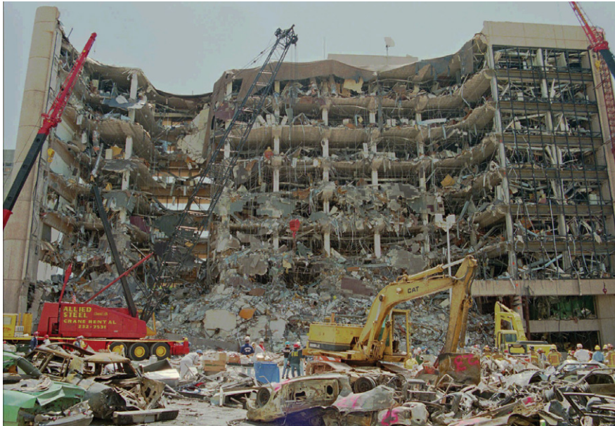
Figure 1.2: Collapse of the Murrah Federal Building. From [2].
