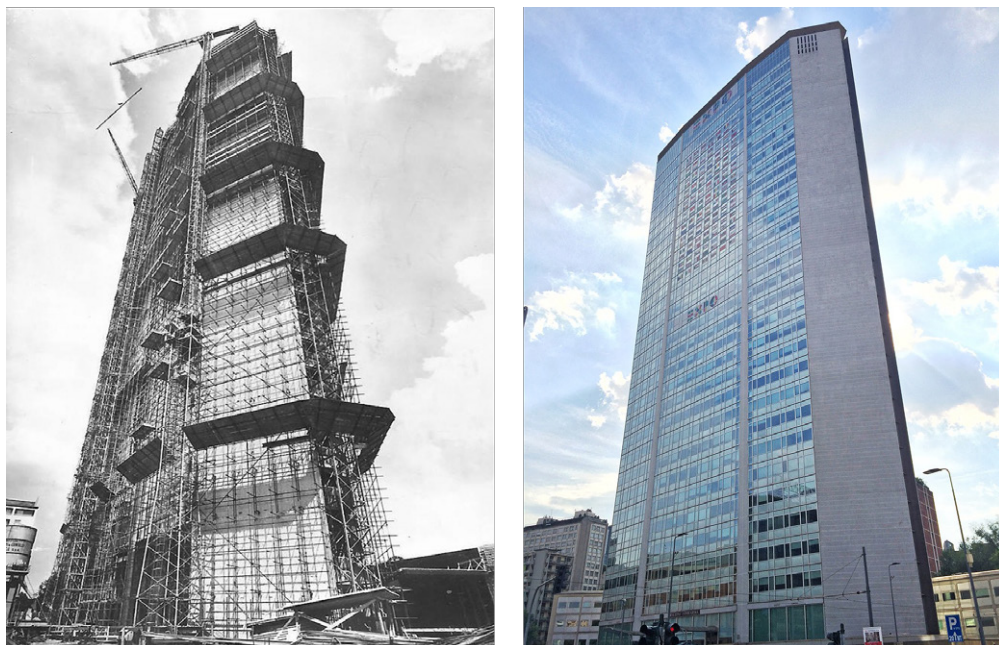
Figure 5.1: Main facade of the Tower during construction (from [33]) and finished (from [7]).
