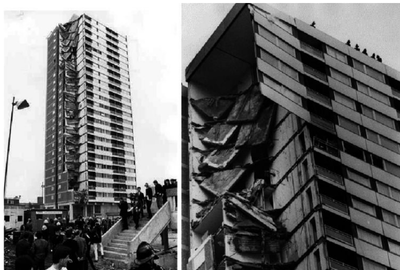
Figure 1.1: Collapse of the south-east corner Ronan Point Tower. From [1].
