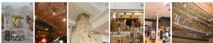
Figure 8. Uncovered structural elements. Source: the authors (2017)
