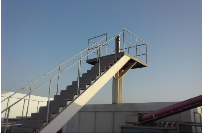
Figure 6. Detail view of Roof station.
