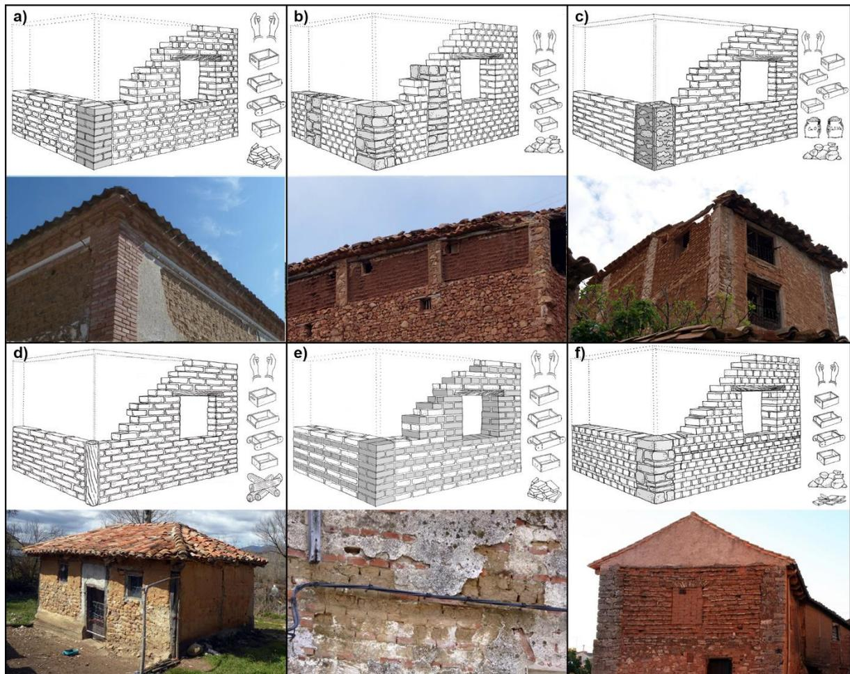
Figure 9. Adobe fabrics in mixed walls (Drawings: SOSierra. Photos: Authors, M. Diodato, L. Villacampa and B. Arnáiz).
