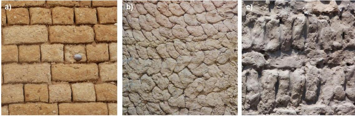
Figure 4. Modelled earthen blocks: a) Adobes; b) Clay lumps; c) Air-dried manual adobes (Authors).
