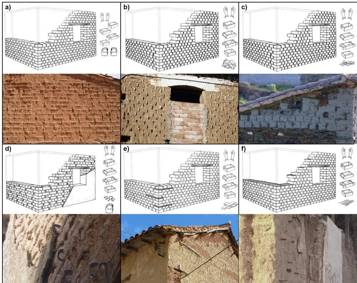
Figure 7. Adobe fabrics with chemical binder layering mortar or insertions in joints (Drawings: SOSierra. Photos: Authors and M. Diodato).
