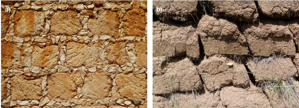
Figure 5. Cut earthen blocks: a) Marl; b) Sod (Authors).
