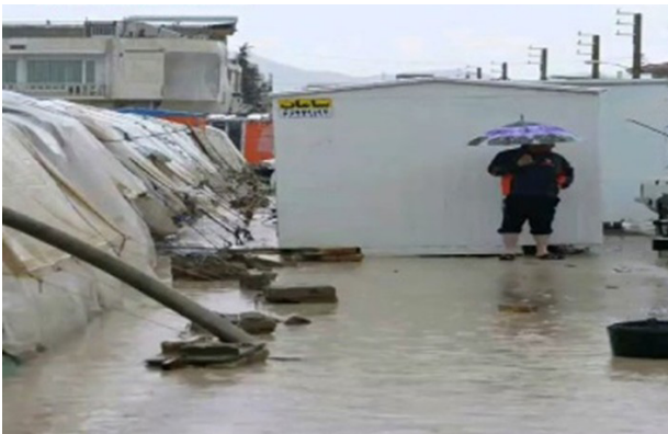
Figure 3. The vulnerability of conventional temporary shelters.
