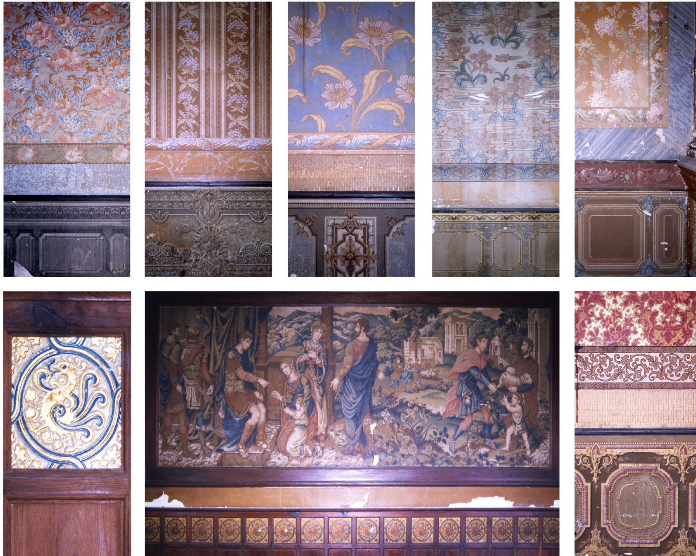
Fig 18. Casa de l'Hort (former Residence-Palace of the Cardinal Payá), Onil (Alicante, Spain), Feb-1996. Photographies of the Initial of the Building before its Drawing and its Rehabilitation. Photographs of the finishes of the noble plan (first floor); top: wallpapers on walls; bottom: wooden or ceramic plinth details. (Original Pictures: Martínez-Medina, A. & Sempere Valero, M.).
