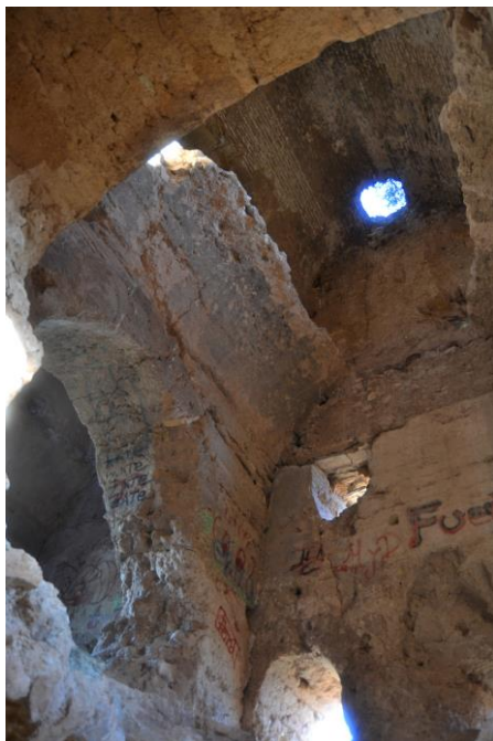
Fig 4. 10 Interior torre Montroi
