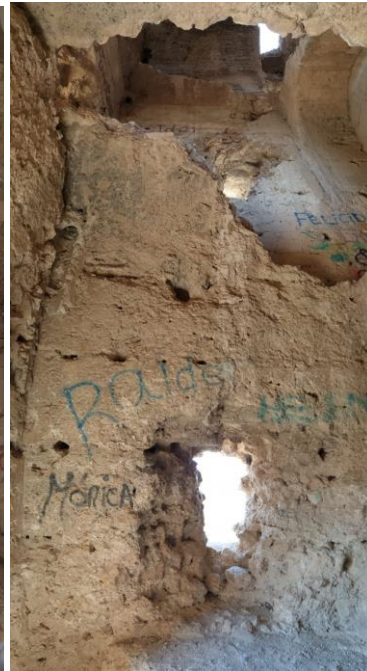
Fig 4. 11 Interior torre Montroi
