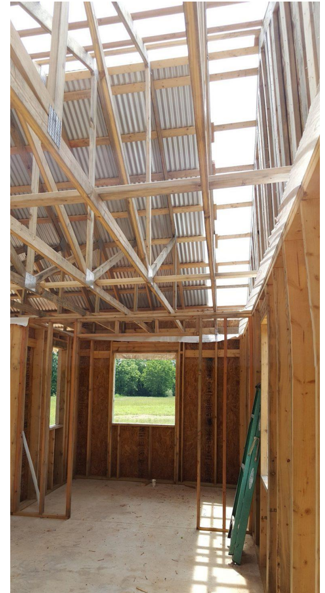
Fig. 186 Buster's Home – Balloon Frame durante la const.
