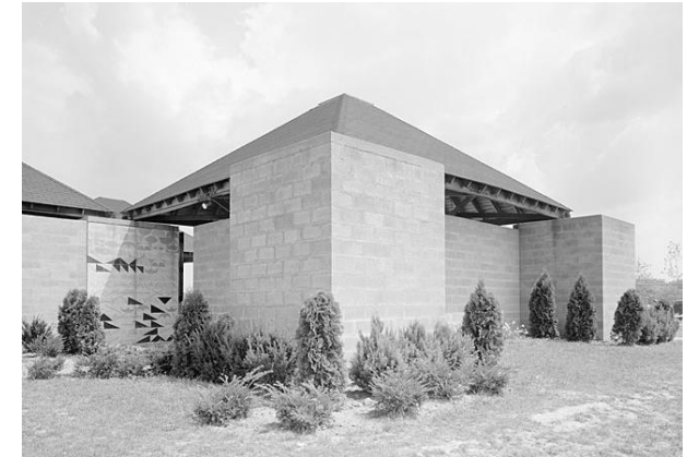
Fig. 21 Kahn - Trenton Bath House - New Jersey, 1955
