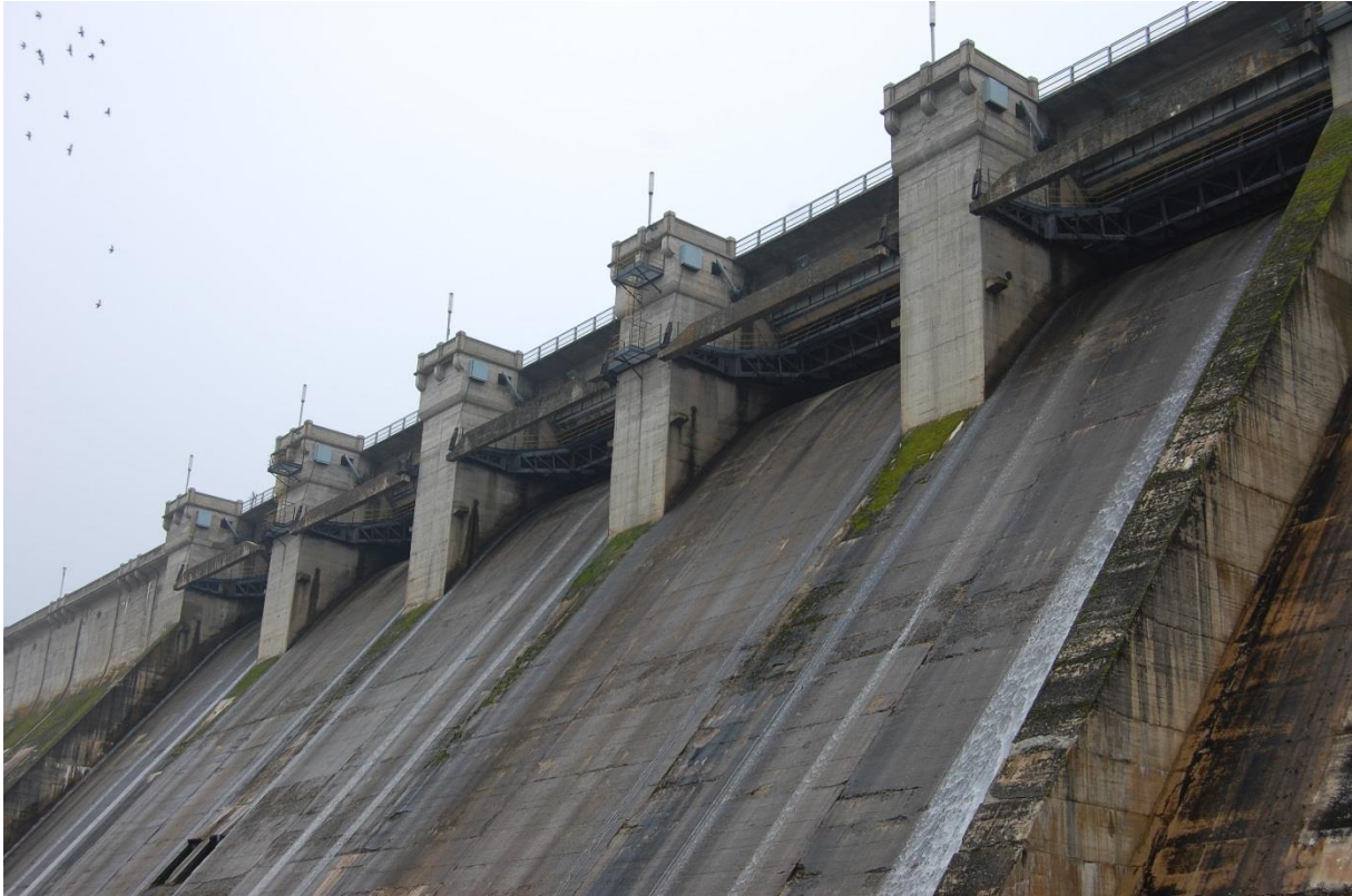
Figure 3. View of the Santa Teresa spillway from downstream.
