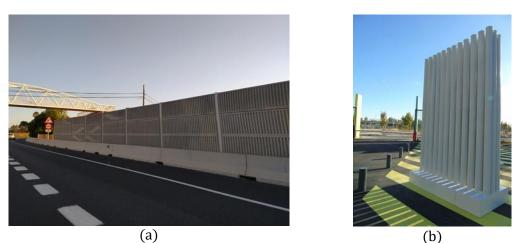
Figure. 32. a) photograph of a traditional continuous noise barrier; b) photograph of a noise barrier based on sonyc crystals concept
