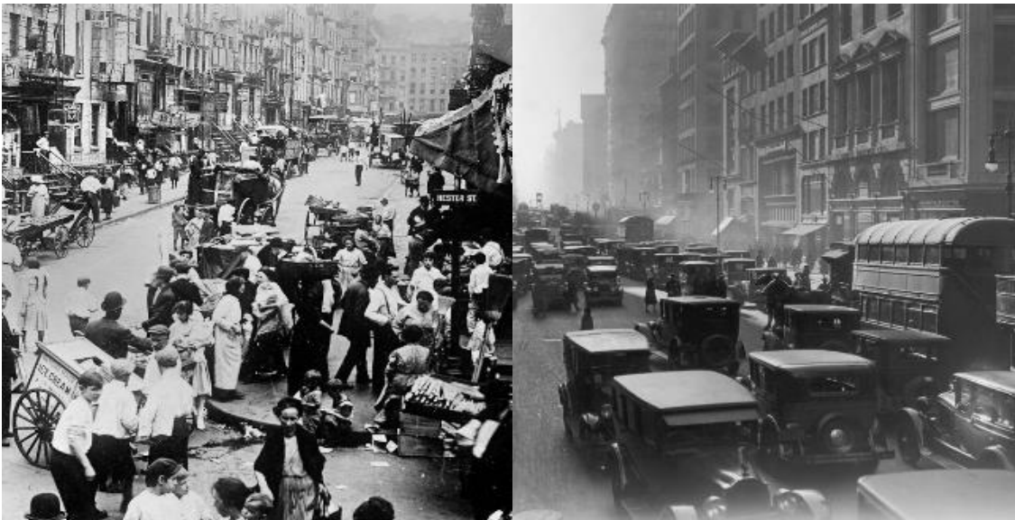
Figure 4: Left: Manhattan's Hester Street, on the Lower East Side, in 1914. (Maurice Branger/Roger Violett/Getty Images). Right: In 1925 Midtown Manhattan, pedestrians compete for space with increasing automobile traffic. (Edwin Levick/Getty Images). Retrieved from: Vox.com
