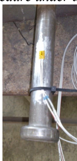
Figure 13. Strain gauge at the mid-height of studs.
