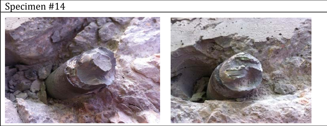
Figure 17. Welding failure in Specimen #14.
