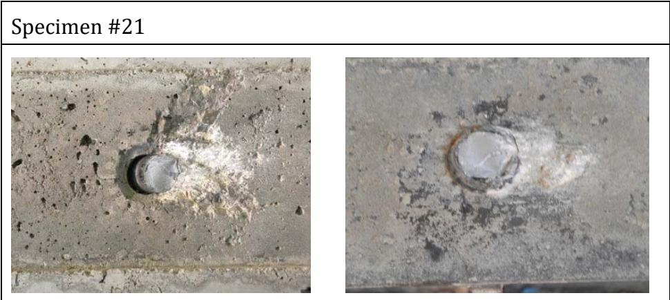
Figure 11. Steel failure in Specimen #21.
