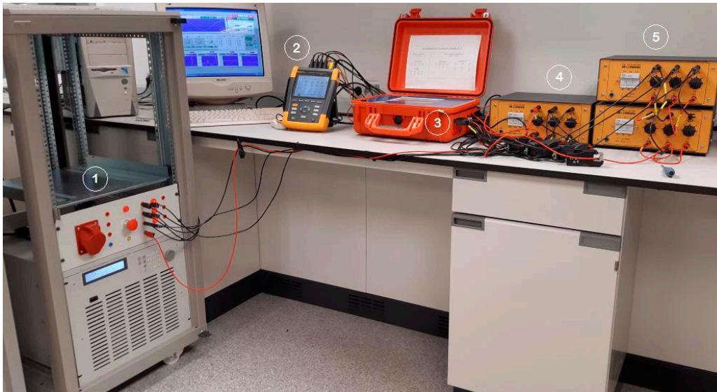
Figure 4. Montage of the testing circuit: (1) Chroma source; (2) Fluke 437; (3) SIMPELEC analyzer; (4) neutral resistances and ammeter clamps; (5) load resistances.
