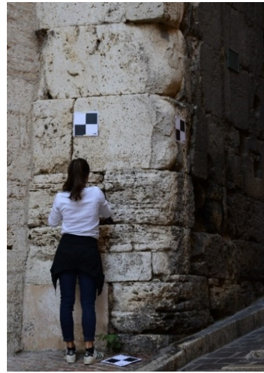
Figure 6: Porta Cornea, detail of the large ashlars.
