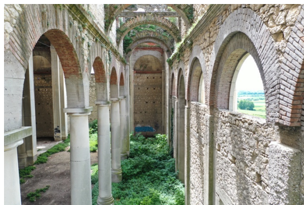
Figure 3: View of the interior spaces of the church after the abandonment.
