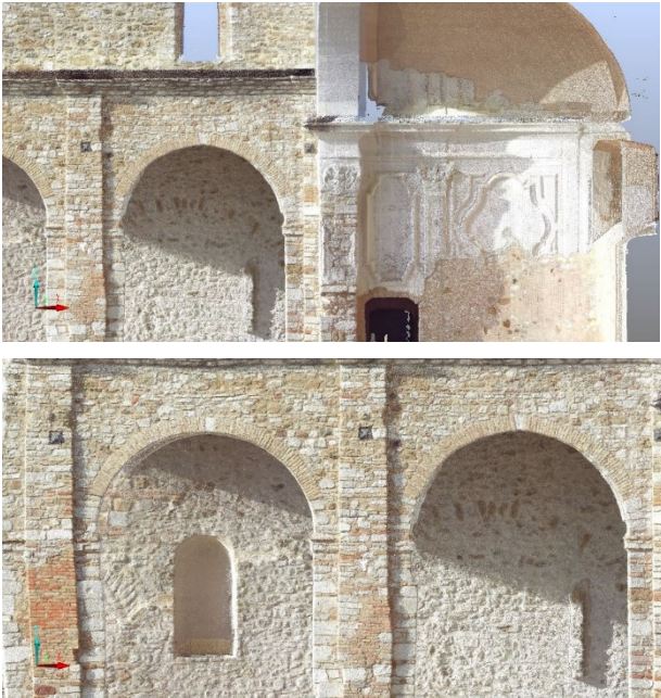
Figure 18: Masonry details of the cathedral. Orthoprojections of the surveyed point clouds.
