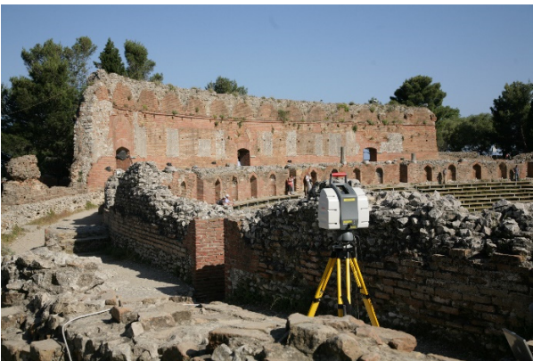
Figure 4: Station from the upper corridor.
