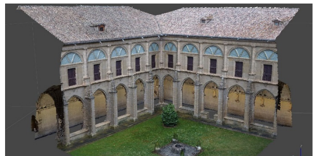
Figure 3: Point cloud of two walls of the cloister from the outside.
