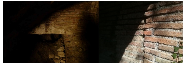
Figure 11: Lower ambulatory of the Amphitheatre. Internal views (R. Marena, October 2019).
