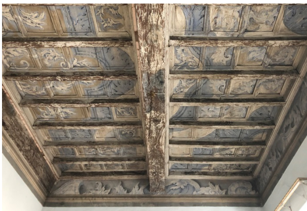
Figure 13: Timber floor in Palazzo Magio with passasotto painting.
