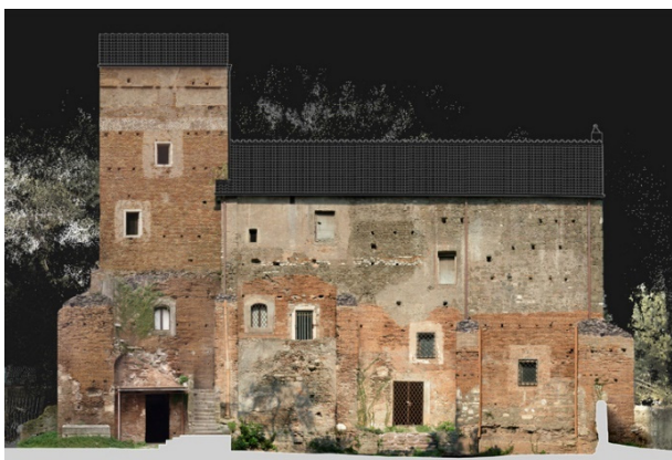
Figure 4: Orthoimage of the southern façade (M. Cola).
