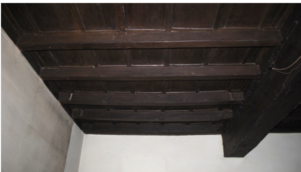
Figure 9: Floor rebuilt at the mezzanine in which the grooves for hosing the bussole are still visible.
