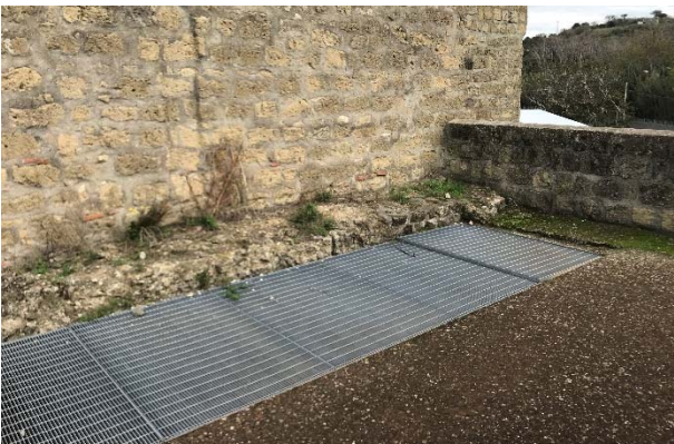
Figure 17: Tempio-Masseria del Gigante, Cuma. The grid for collecting rainwater on the terrace.
