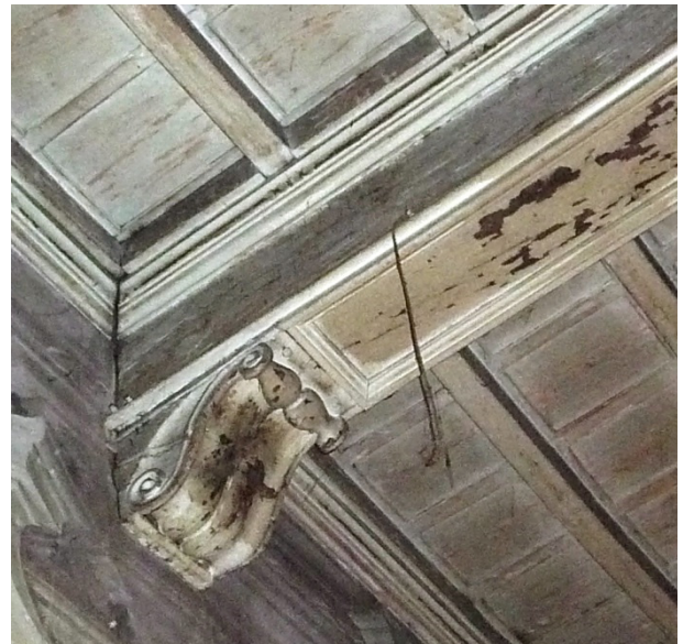
Figure 7: Detail of the floor in fig. 6.
