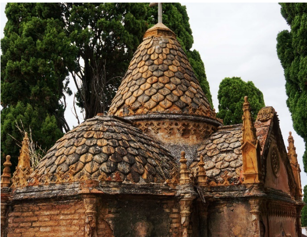
Figure 4: Terracotta roof tiles: the two different colours that form a geometric pattern are still visible despite the decay of the surface.
