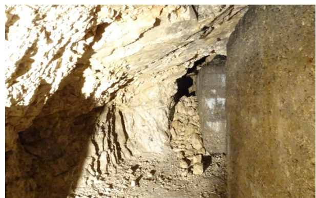
Figure 4: View of vault collapse within the infirmary tunnel.
