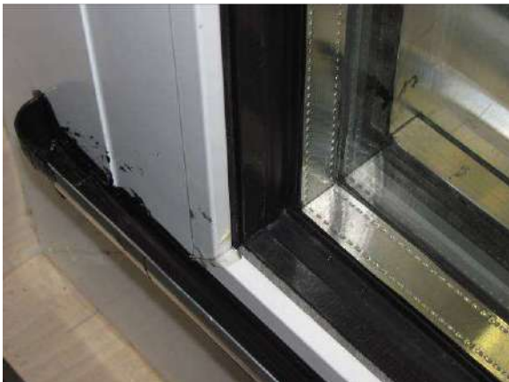
Photo 7 Internal sash, FR 1 at bottom lock side
