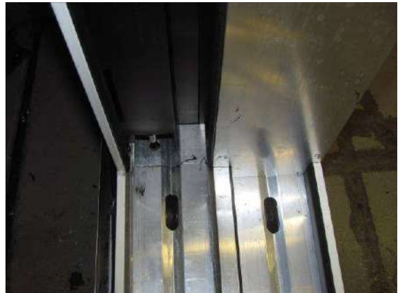
Photo 3 Internal rebate seal at bottom, corner design at bottom lock side FR 1
