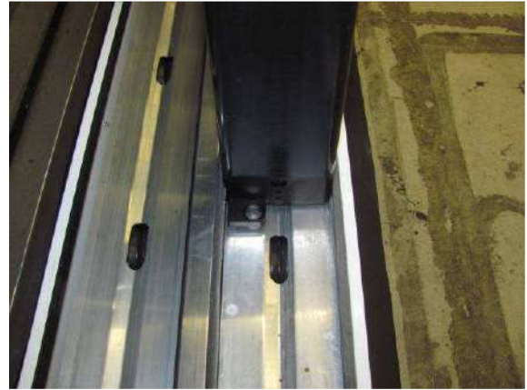
Photo 11 Locking situation sash
