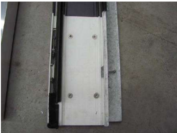
Photo 4 Coupling profile Item No. 460430 with flat steel, central seal and centred area seal
