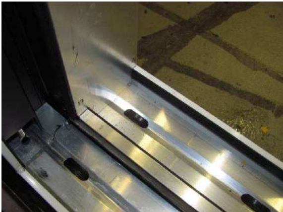
Photo 2 External rebate seal, at bottom, corner design at bottom lock side FR 1
