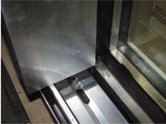
Photo 5 Coupling profile with flat steel and sealing cap (FR 1 internal at bottom)
