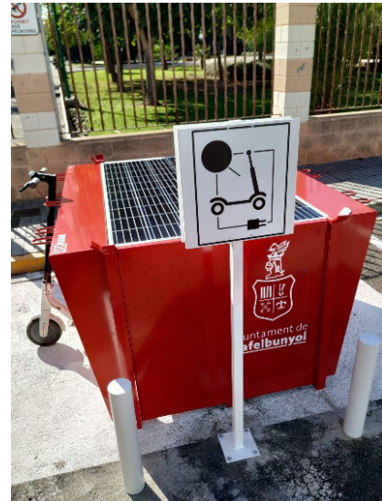
FIGURE 1. PV-based e-scooter recharging dock installed near a public park in Rafelbuñol.
