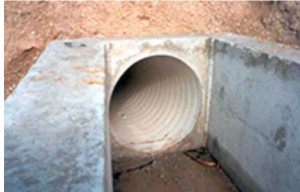
Figure 2. PVC pipe for diameters of more than 1200 mm. Source: RIBLOC
