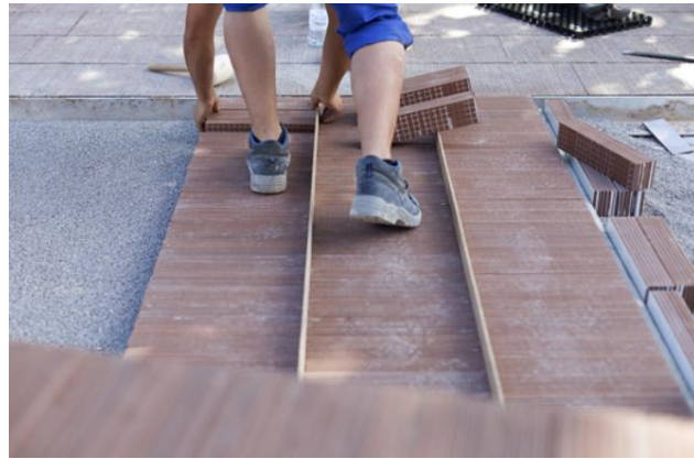
Figure 18. Disposition of ceramic on Benicassim, Castellon. Source: Life CERSUDS
