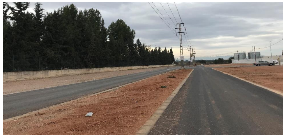
Figure 15. Beginning of the improvement of Calle Sequia de Mislata, catchment N1
