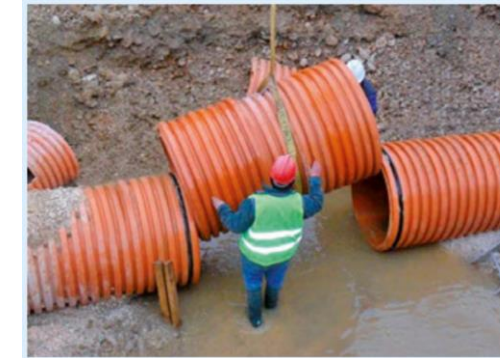
Figure 1. PVC pipe for diameters of less than 1200 mm. Source: SANECOR
