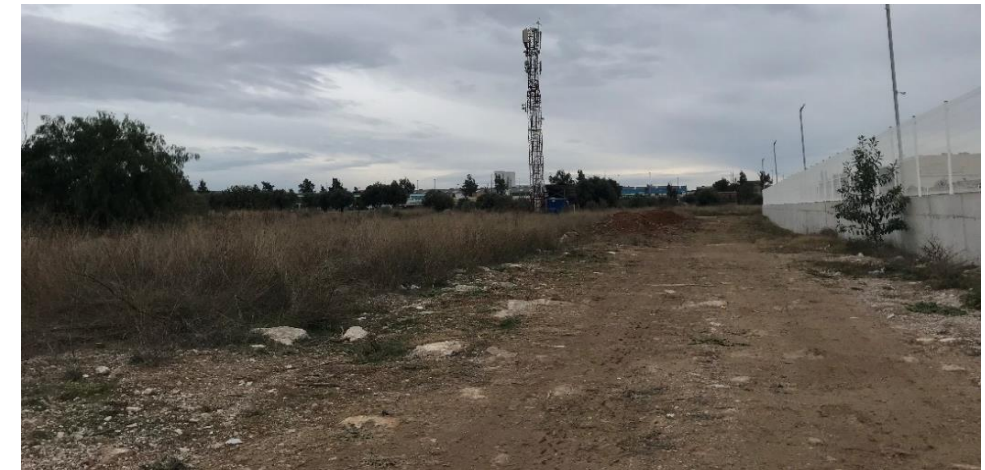
Figure 11. Road status Calle Polígono 13, catchment N1
