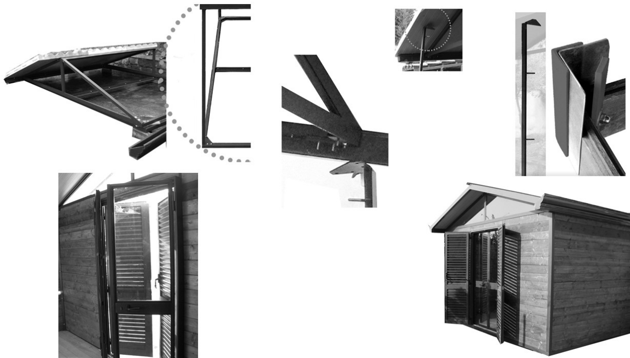
Figure 4 | The system with the vertical assembly and the mounted slats.
