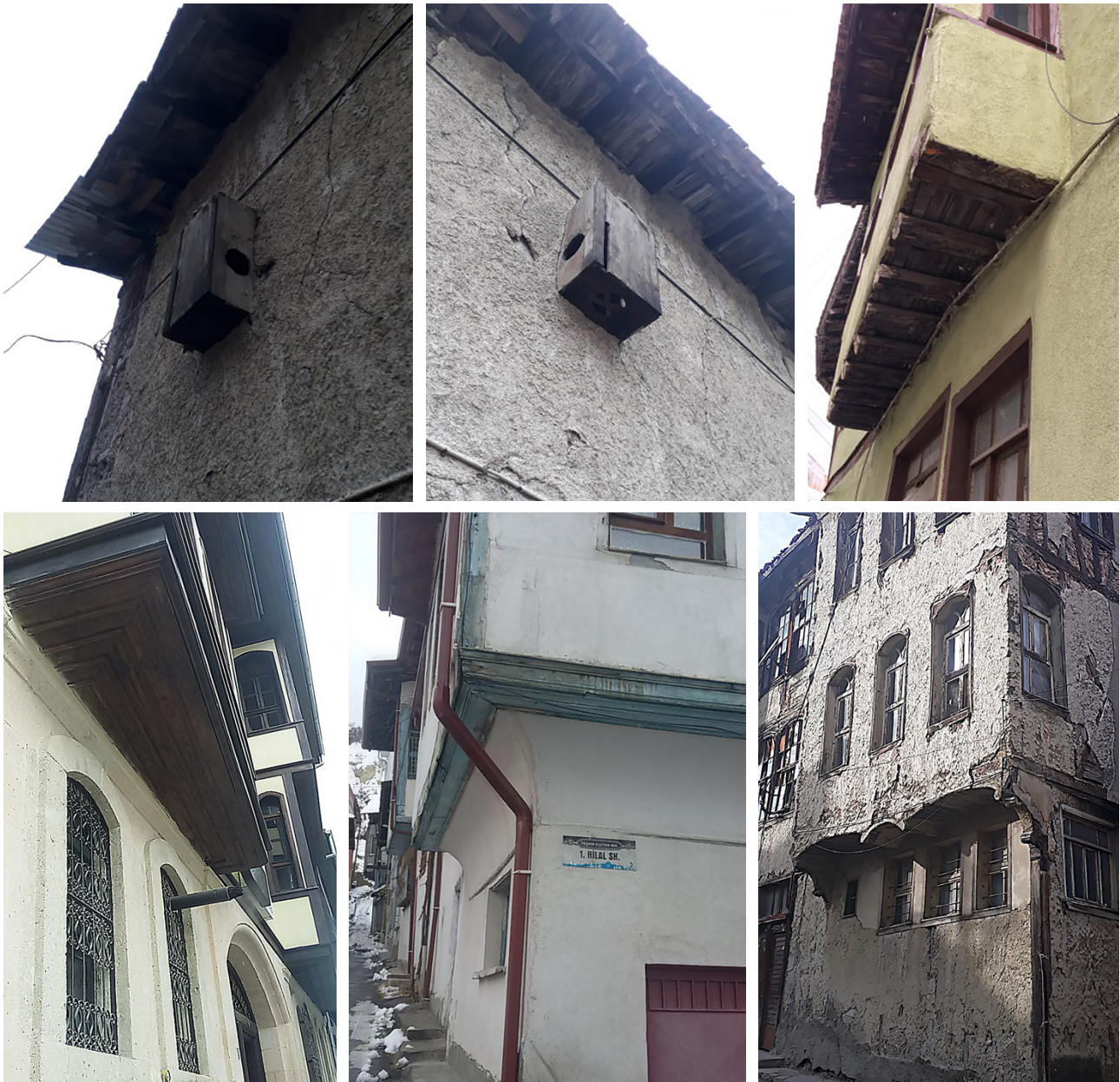
Figure 2 | Views from “süt dolabı” in a traditional Kutahya house (top), and types of protrusion areas in living spaces; carried on floor beams (top-right), with flat coated (bottom-left and center) and coated with curved ornaments (bottom-right)
