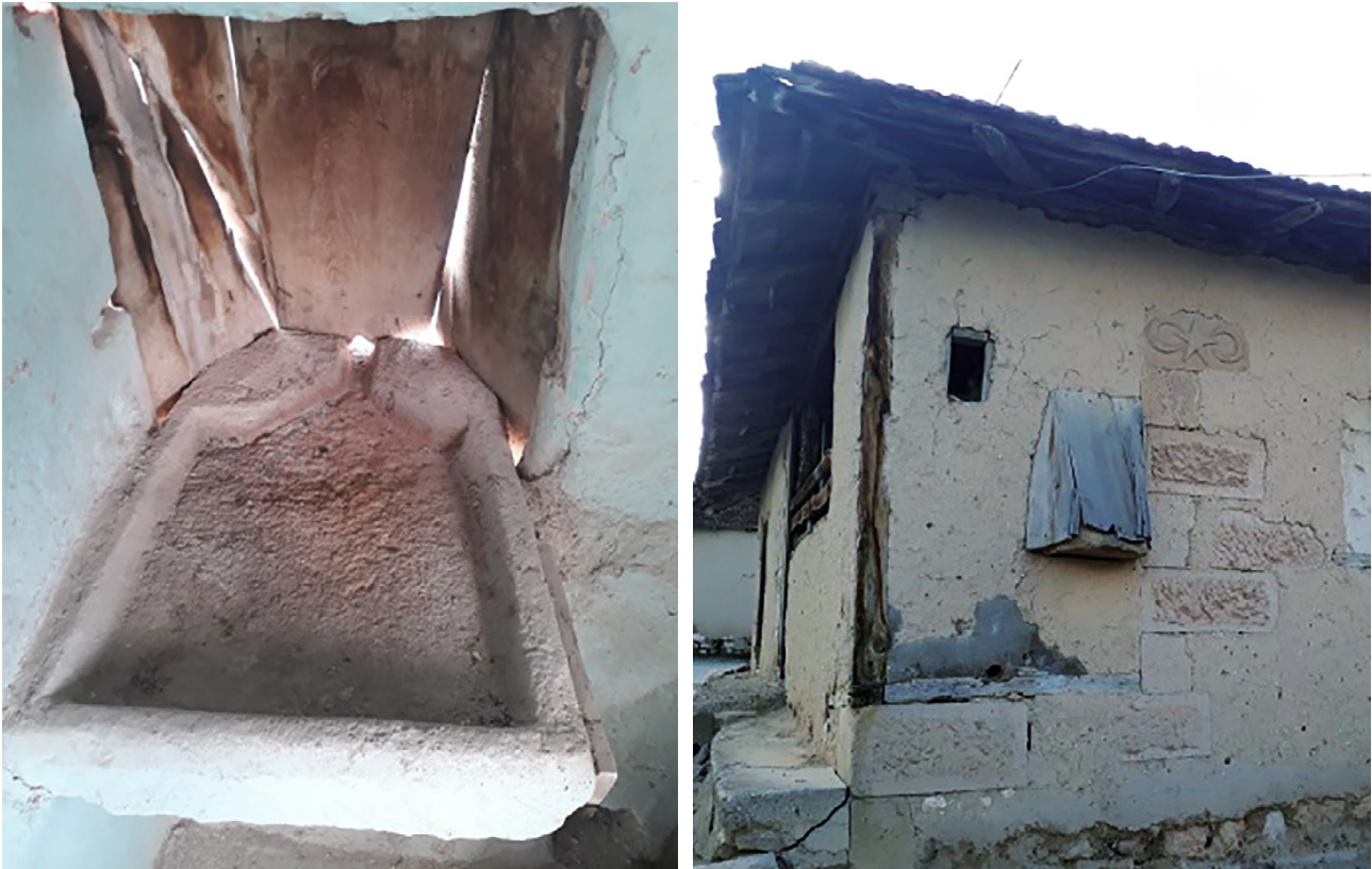
Figure 1 | Interior (left) and exterior (right) views of an original ablution space protruded from the facade (a guesthouse in Siner Village, Kutahya).
