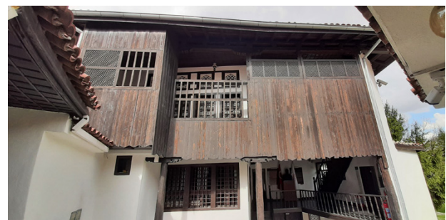
Figure 14 | Views from the large wooden eaves, downspouts, downpipes, and tile covering (top and bottom).
