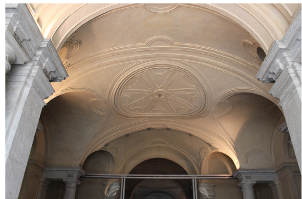
Fig. 3. Palazzo Mazzonis' vaulted atrium (Source: own's).
