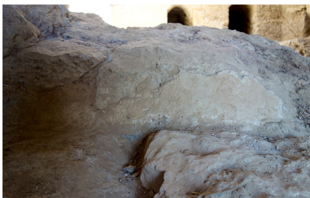
Figure 6. White mortar at the bottom of the wall.
