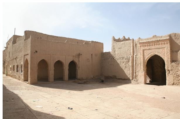
Figure 9. Square located in the access to the interior of the Oulad el Haj Ksar (22EP), in which the facilities for community use are located. Source: Gil-Piqueras & Rodríguez-Navarro.
