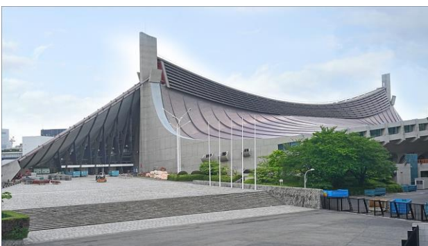
Figure 13. Yoyogi National Gymnasium. Photography Jean-Pierre Dalbéra.
