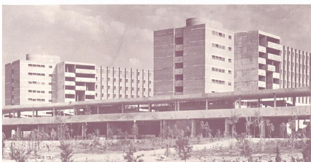
Figure 2. Residences area. Architecture 142, 1970.
