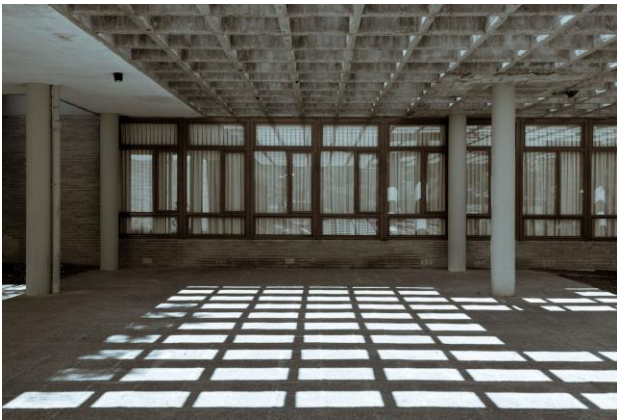
Figure 5. President's office. External louvers. Photography Ximo Michavila.
