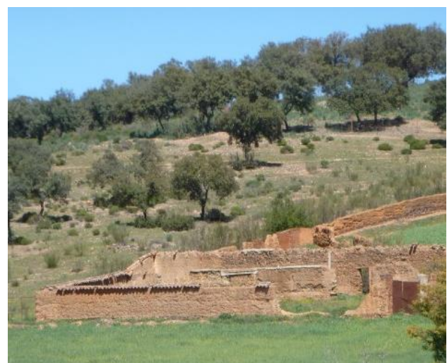
Figure 1. Relationship between the matter from the landscape and the rammed earth walls (Navalpino, Ciudad Real)
