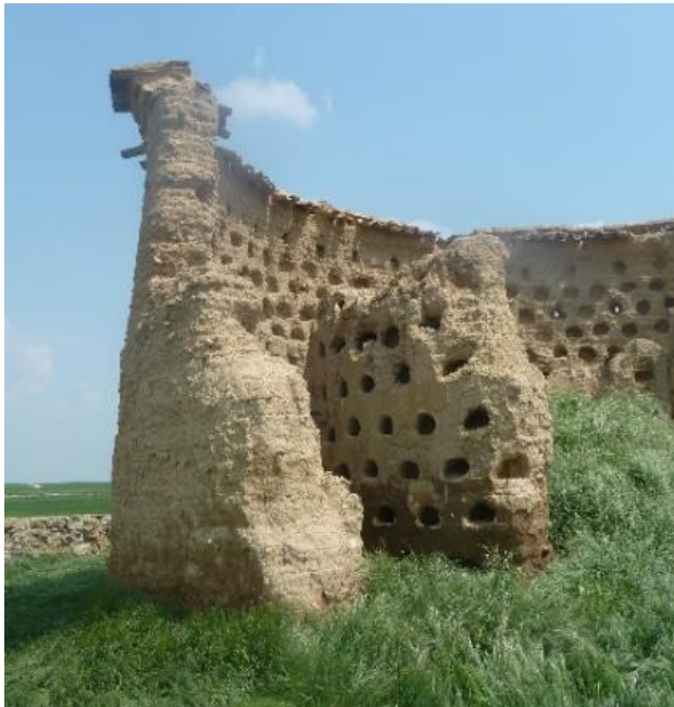
Figure 2. Abandonment by functional obsolescence of earthen architecture (dovecote in Castilla y León)
