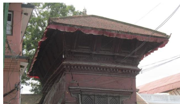
Figure 1. Effects caused by 2015Ghoroka earthquake.
