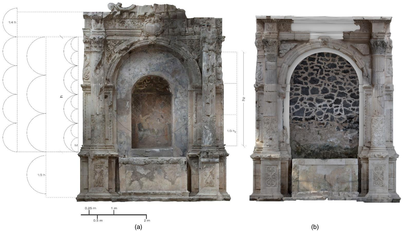
Figure 11: a) 3D model of the altar of Sant'Erasmus; b) 3D model of the altar of the Purgatorio. In white, NURBS.n the original colours, photogrammetric mesh of the surviving parts.
