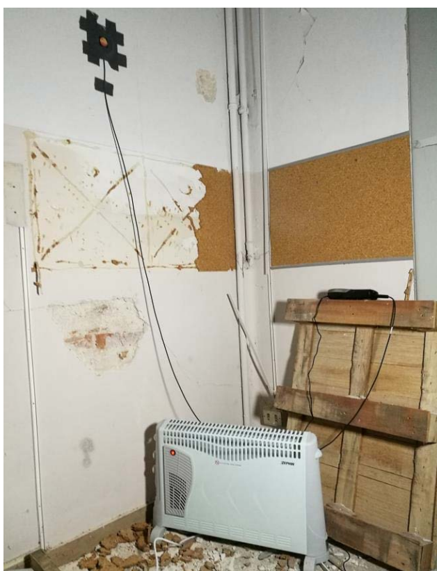
Fig. 16: The plate on the inner side of the masonry to analyse
