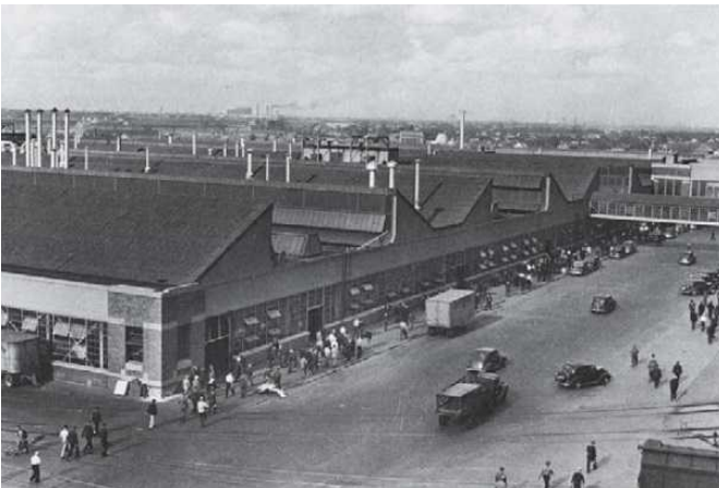
Fig. 71. Ford River Rouge Assembly Building (1925)
