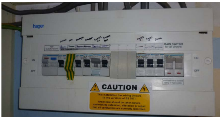
Figure 31 Electric Circuits Control
