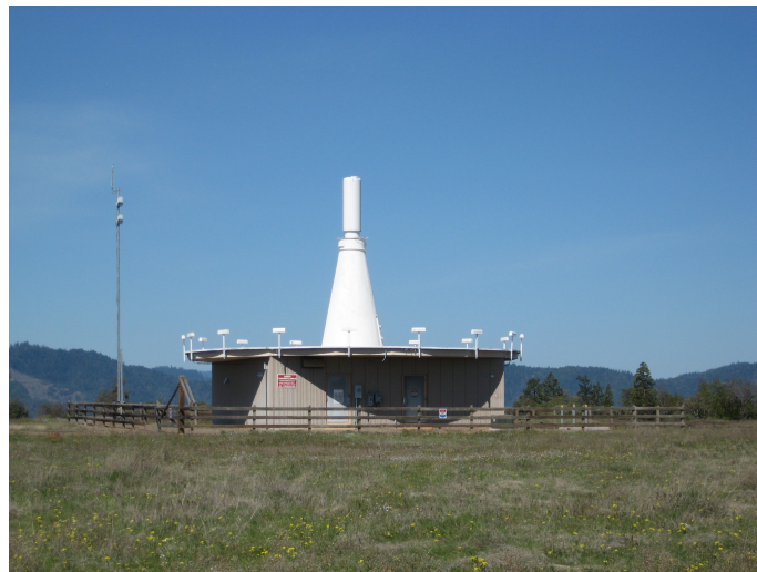
Figura 9. Ground Station of a VOR [3]
