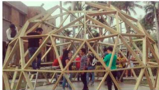
(a) Details of the geodesic dome at the University of Magdalena.
