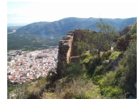
Fig. 38 Vista interior torre sureste
