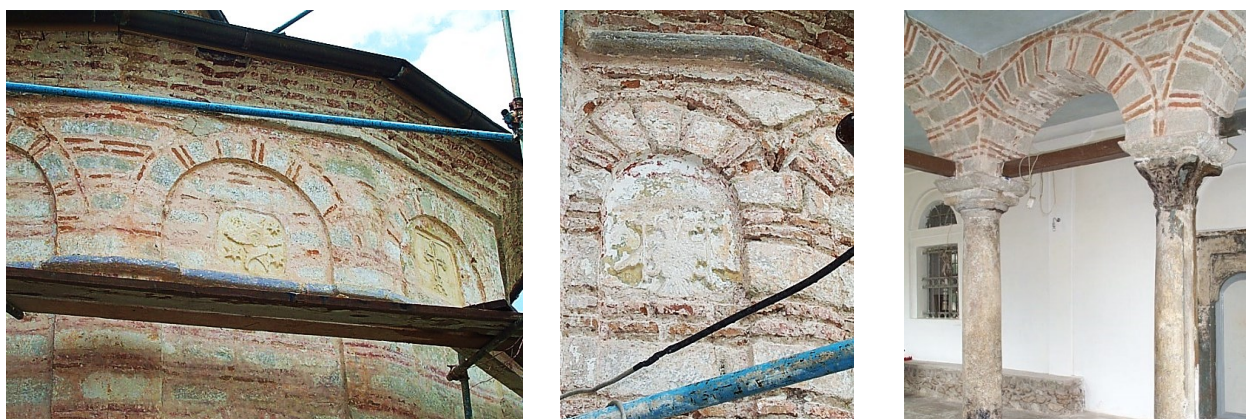
Figure III.235 St. Demetrius in Bitola. Details of shallow reliefs: A-B. Details of the altar apse; C. Spoliae in the southern porch.
