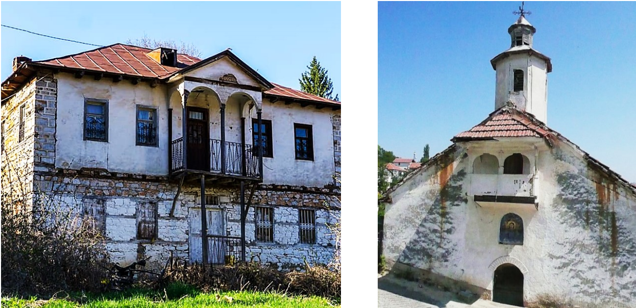
Figure III.36 Comparison between Revival wooden balconies: A. Main façade of a house in the village of Prostranje, near Kichevo; B. Western façade of the church of St. Savior in Rogachevo (Tetovo).
