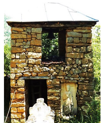
Figure III.94 The bell tower of St. Archangel Michael in Kokre (Mariovo).
