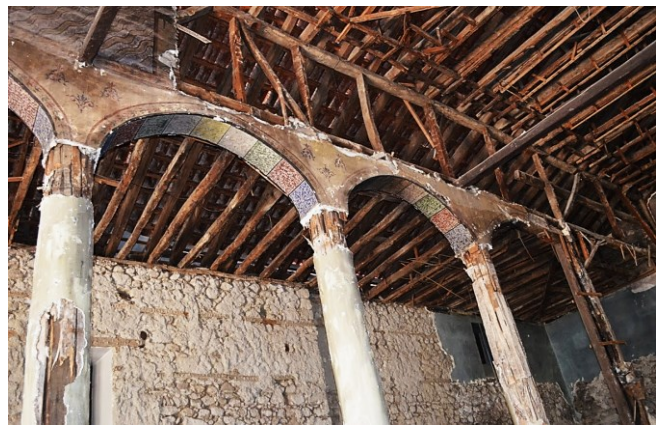
Figure III.11 Examples of "false" wooden vaults and flat ceilings. A. St. Savior in Gabrevci (Radovich); B. St. Demetrius in Kavadarci.
