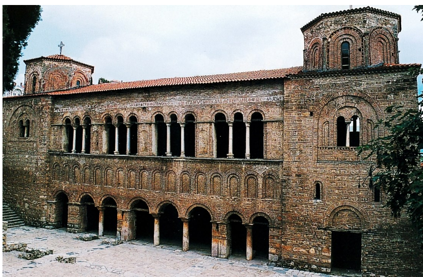
Figure I.24 The exo-narthex of St. Sophia in Ohrid, added in the early XIV century.
