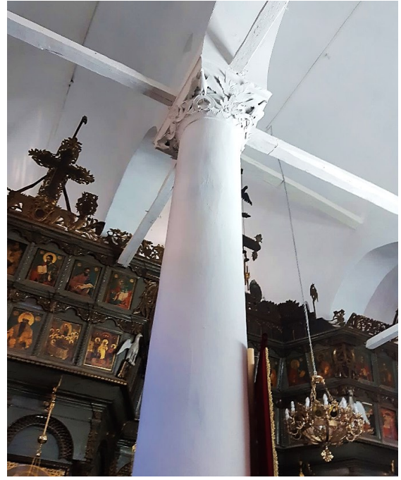
Figure III.101 Details of wooden columns and wooden ( kjulum ) capitals: A. St. Demetrius in Kriva Palanka; B. St. John in Kratovo.
