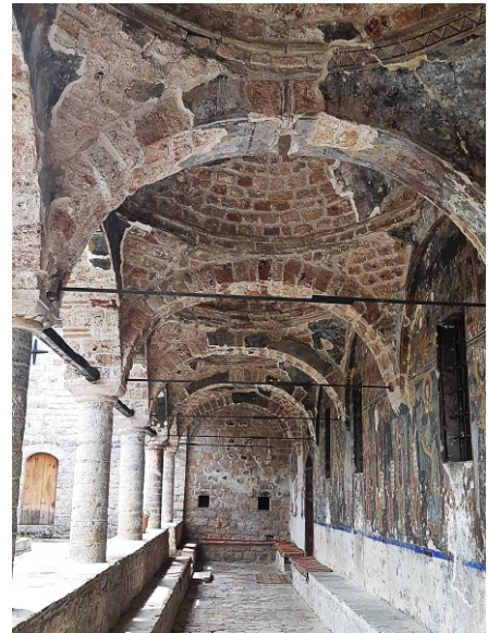
Figure II.6 The southern porch of St. Nicholas in Moskopole (Albania).
