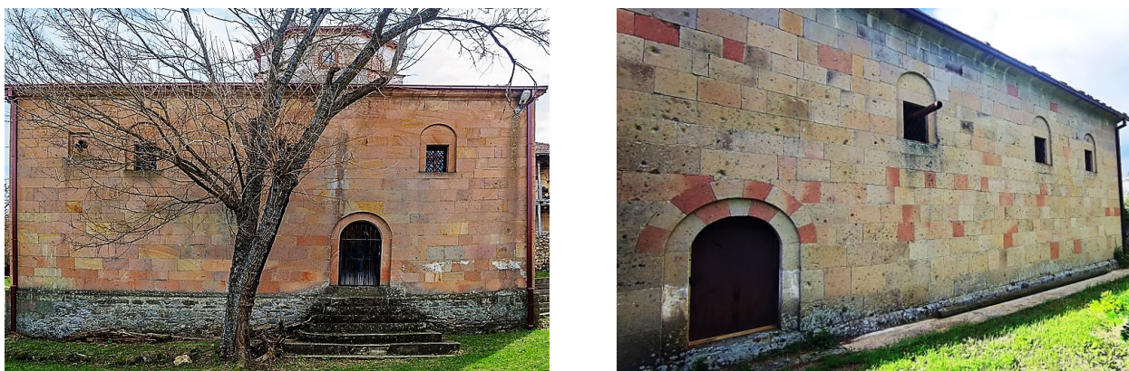
Figure III.5 A. The northern façade of the Zabel Monastery , near Kumanovo; B. The southern façade of the church of St. Demetrius in Stracin (Kratovo).
