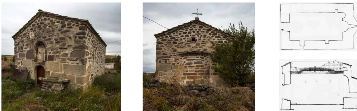
Figure I.42 Post-Byzantine vaulted single-nave churches: St. George in Gjumelci (Sveti Nikole). View from the southwest and east; plan and longitudinal section.
