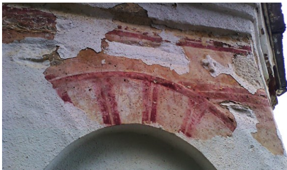
Figure III.6 St. Demetrius in Bukovo (Bitola). Detail of the painted masonry opus on the altar apse façade.
