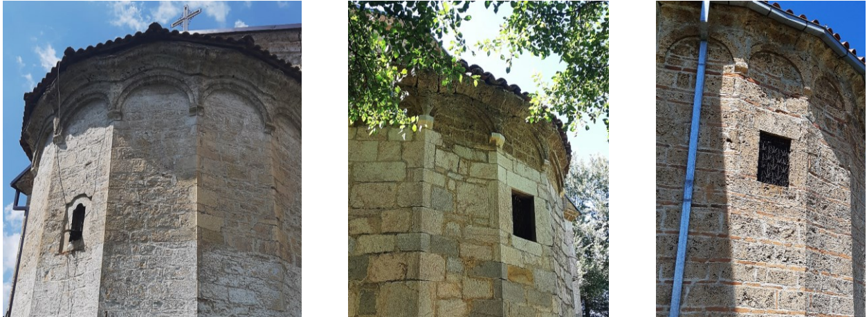
Figure III.28 Examples of altar apses with a frieze of cantilevered arcades: A. St. George in Resen; B. St. Nicholas in Carev Dvor and C. St. George in Drmeni, all in the region of Prespa.
