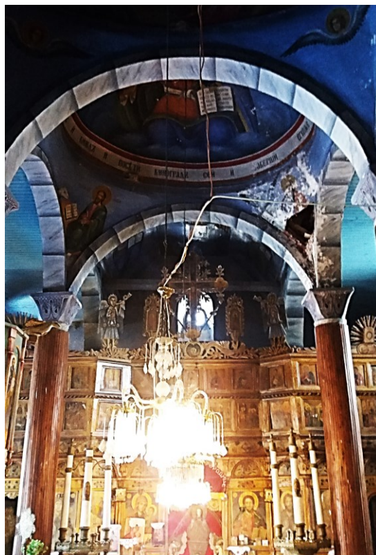
Figure III.14 The Most Holy Mother of God in Duf (Gostivar). View of the false blind dome in the central nave and its wooden substructure.
