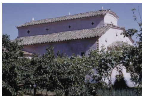
Figure III.205 St. Savior in Drachevo (Skopje) in 1954. View from the south-east.
