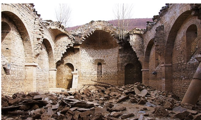
Figure III.10 Interior view of the church of St. Nicholas in Mavrovo, after 70 years of submersion in the artificial lake Mavrovo.
