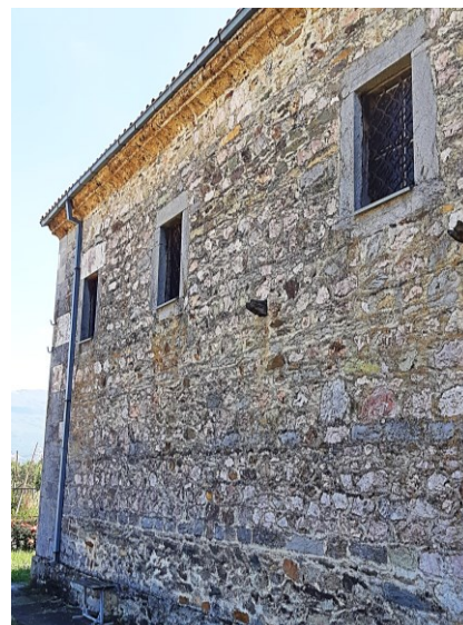
Figure III.184 St. George in Drmeni (Prespa). Detail of the northern façade.
