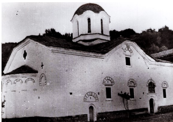
Figure III.215 St. Sotir in Bukovo (Bitola), photographed in 1899. View from the north-east.
