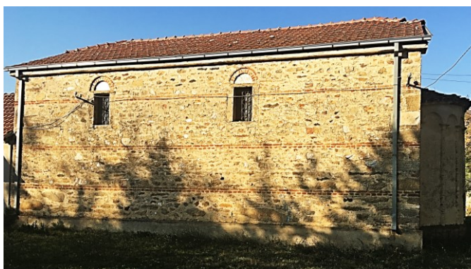
Figure III.7 St. Athanasius in Senokos (Prilep). Horizontal leveling layers of the façade, executed in brick. View from the southeast.
