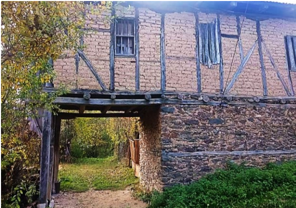
Figure III.9 Examples of vernacular architecture. Use of combined construction systems: massive stone masonry with visible wooden braces and wooden frame with adobe brick infill. A: village of Vrbjani B: village of Mramorec.
