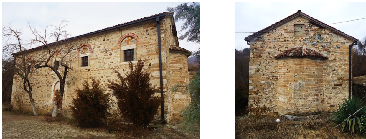
Figure III.125 St. Savior in Creshevo (Skopje): A. View from the southeast; B. East façade.
