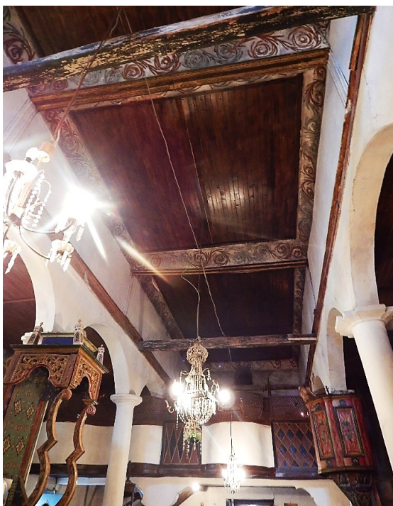
Figure III.105 Details of flat wooden ceilings: A. St. Nicholas in Bashino Selo (Veles); B. St. Elijah in Blatec (Vinica).
