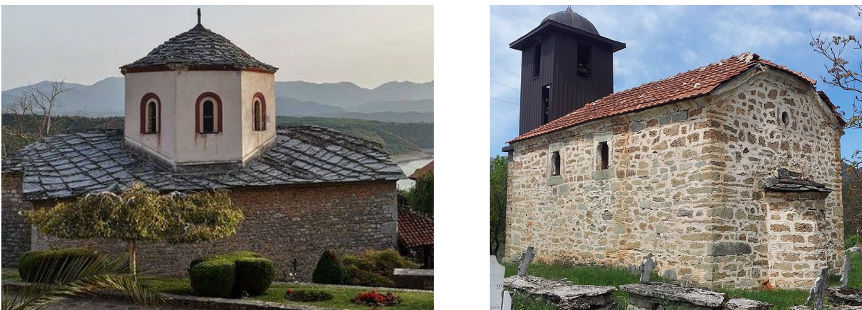
Figure III.15 Examples of partially or entirely preserved stone-slab roofs: A. St. George in Rajchica (Debar); B. St. Savior in Trebovlje (Makedonski Brod).
