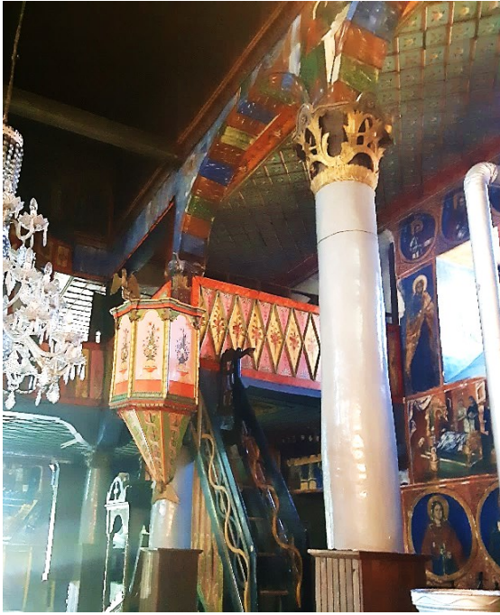
Figure III.101 Details of wooden columns and wooden ( kjulum ) capitals: A. St. Demetrius in Kriva Palanka; B. St. John in Kratovo.
