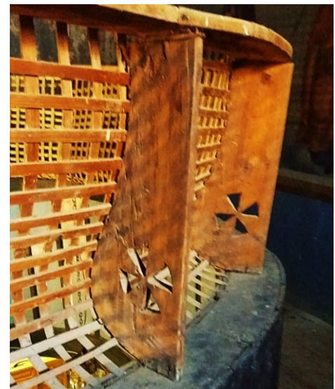
Figure III.41 Examples of musharabia railings, placed above the gallery parapet: A. The Most Holy Mother of God in Krushevo; B. The Most Holy Mother of God in Duf (Gostivar).
