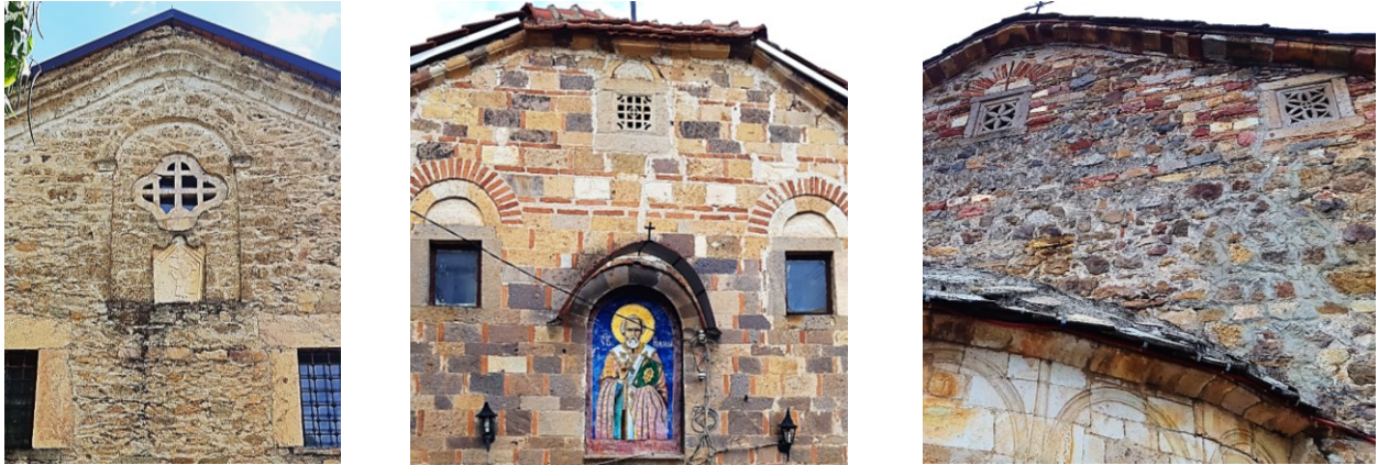
Figure III.77 Transennas with a complex design: A. St. George in Resen; B. St. Nicholas in Kratovo; C. St. John in Kratovo.
