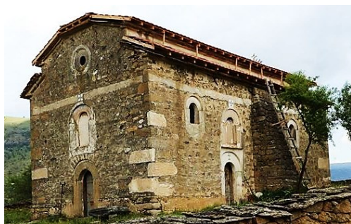
Figure III.145 St. Savior in Kalen (Mariovo). View from the south-east and south-west.
