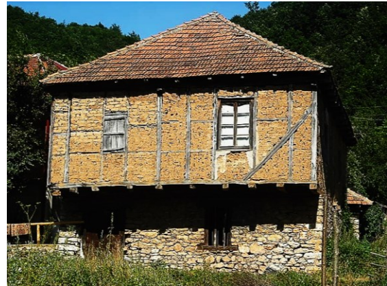
Figure III.9 Examples of vernacular architecture. Use of combined construction systems: massive stone masonry with visible wooden braces and wooden frame with adobe brick infill. A: village of Vrbjani B: village of Mramorec.
