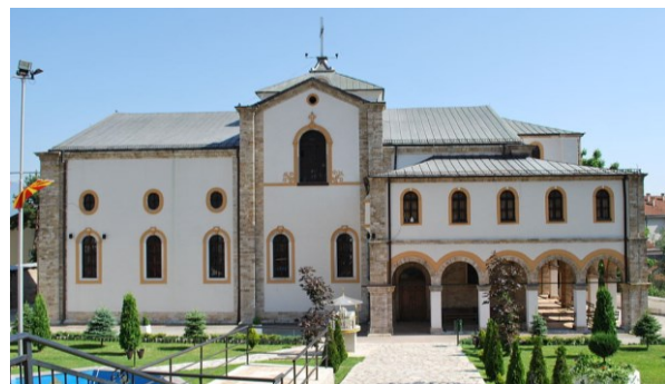
Figure III.264 St. Cyril and Methodius in Tetovo. View from the north.
