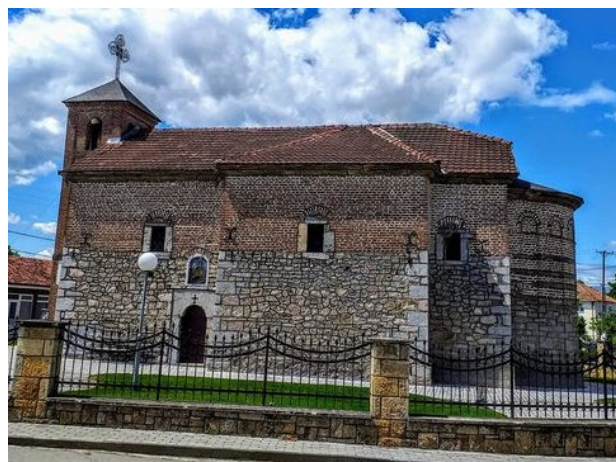
Figure III.256 Examples of single-nave basilica / trefoil combined solutions with blind domes: A. St. Archangel Michael in Vrutok (Gostivar); B. St. John the Baptist in Mislehevo (Struga).
