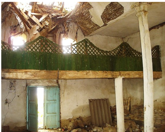
Figure III.11 Examples of "false" wooden vaults and flat ceilings. A. St. Savior in Gabrevci (Radovich); B. St. Demetrius in Kavadarci.
