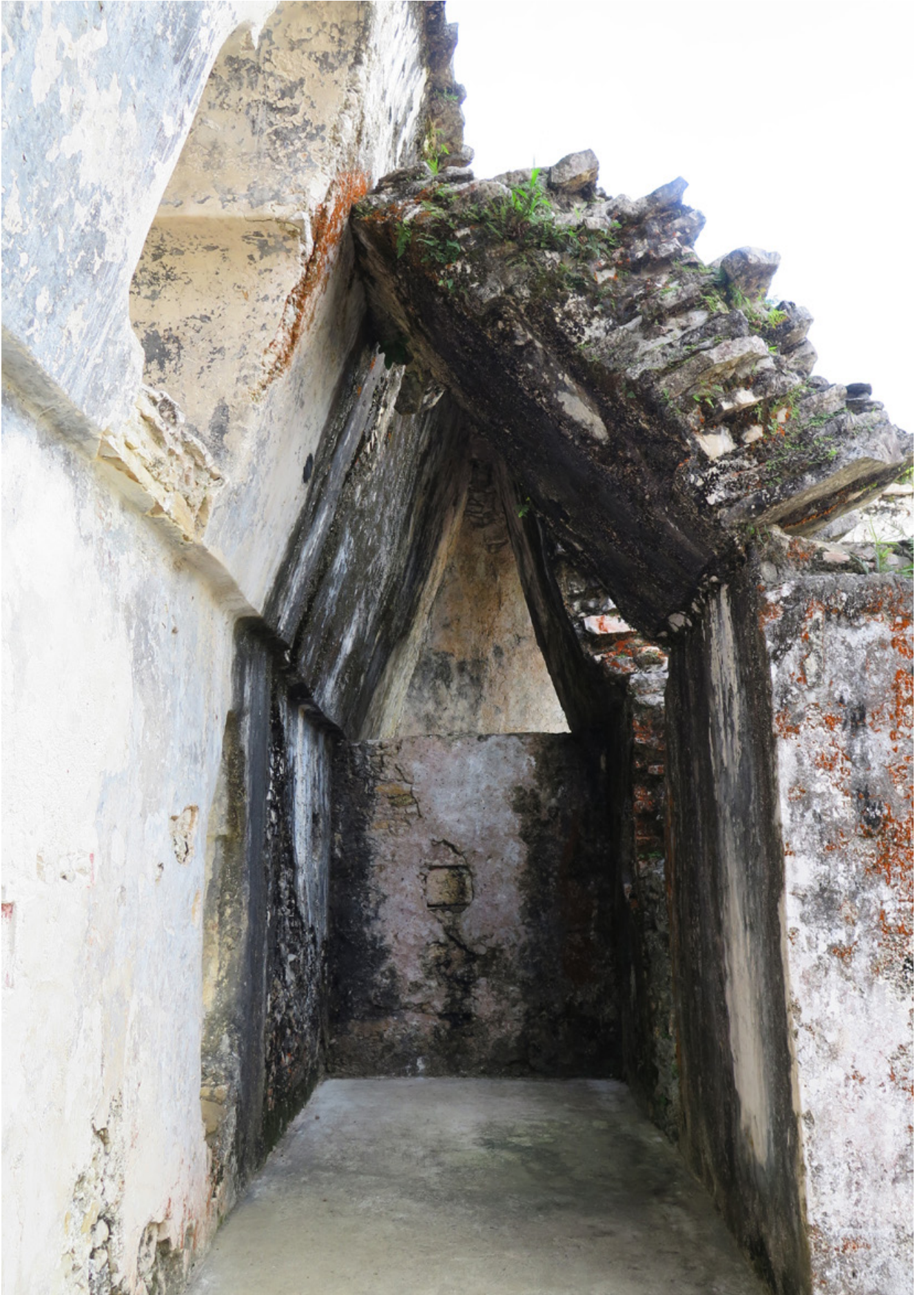
Fig. 17: Collapsed vault in the Palace of Palenque
