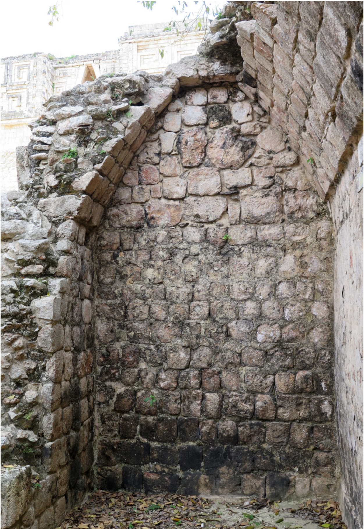
Fig. 15: The change in end-vaults stones bond indicates two differentiated phases of the building process in Chenes Building 1 in Uxmal
