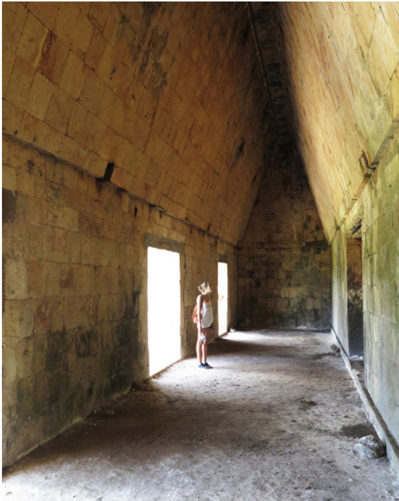
Fig. 16: Vaulted room of the House of the Governor in Uxmal
