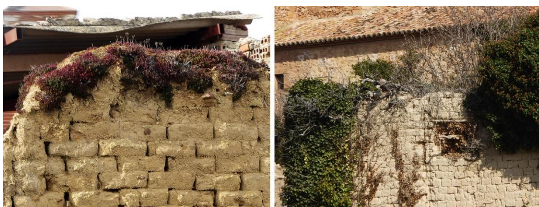
Figure 11. Proliferation of mould and lichen (left) and vegetation growth (right).
