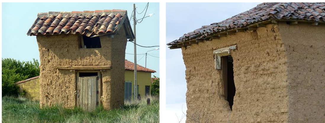
Figure 9. Erosion through the action of the wind.
