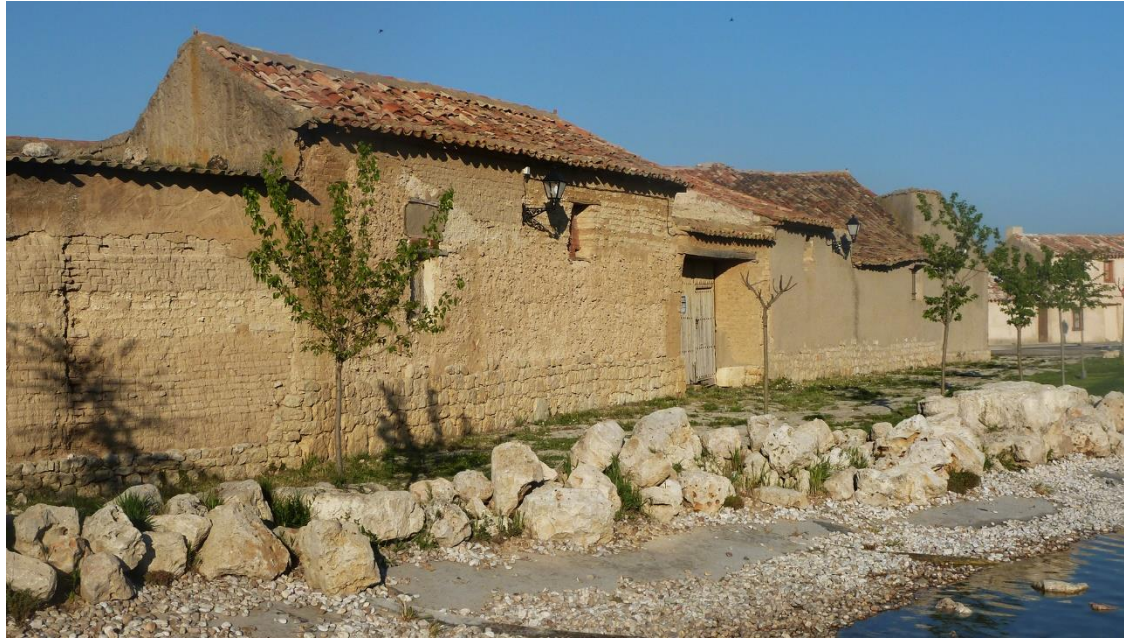
Figure 1. Adobe constructions in Uruña, Valladolid.
