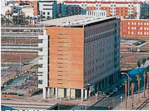
Ref. 4.31. Vista general
