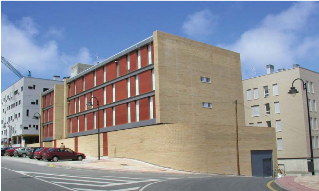
Ref. 4.162. Fachada principal
