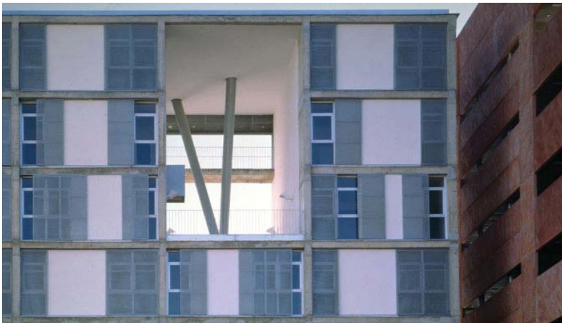
Ref.4.119. Fachada interior
