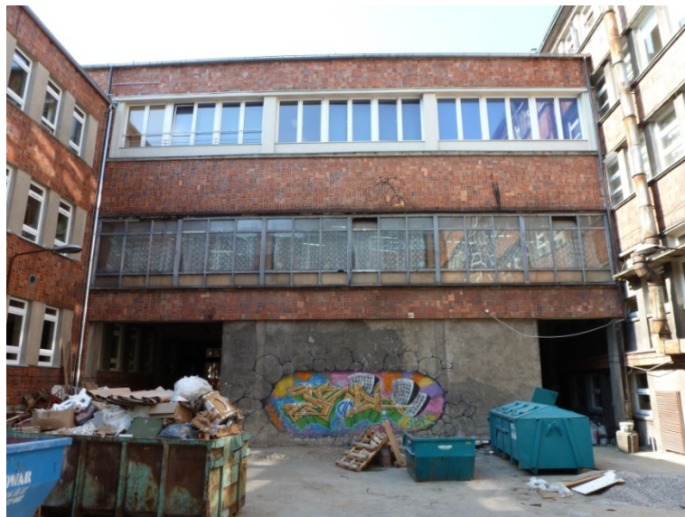
Fig. 5.9. Library north view (done by R.F.P)
