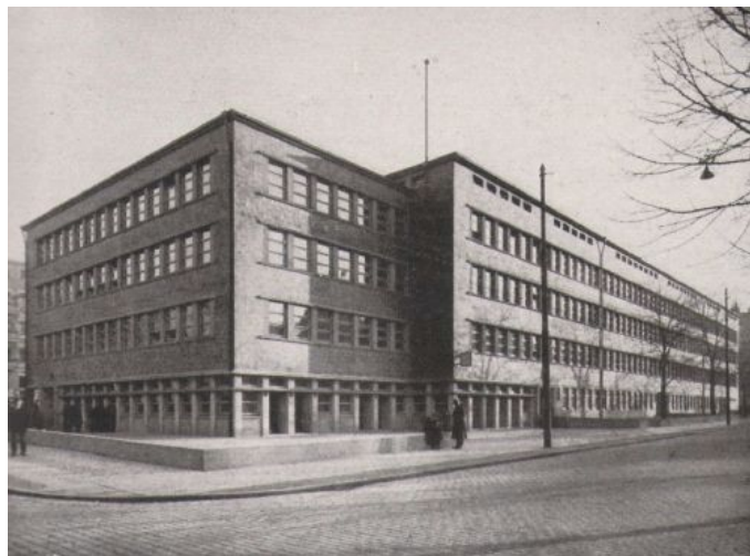
Fig. 3.2. Faculty of Civil Engineering and Architecture building (1939) [2]
