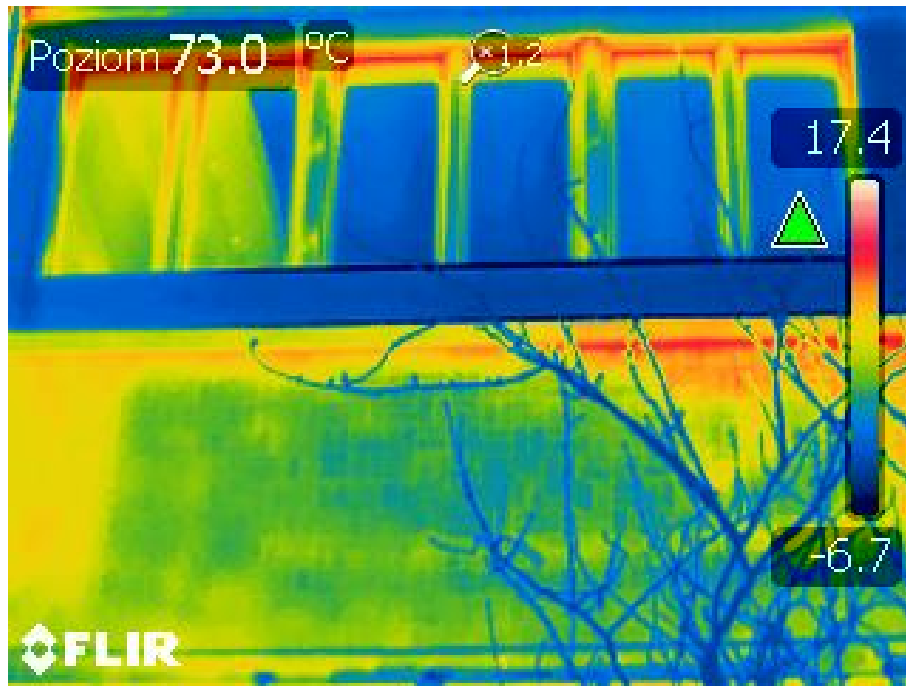
Fig. 5.16. Library south view, thermography 6 (done by R.F.P.)
