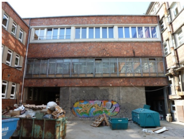
Fig. 4.5. North view of the library from the courtyard (done by R.F.P.)
