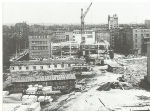
Fig. 4.1. Construction of the Faculty of Civil Engineering and Architecture (1965) [3]
