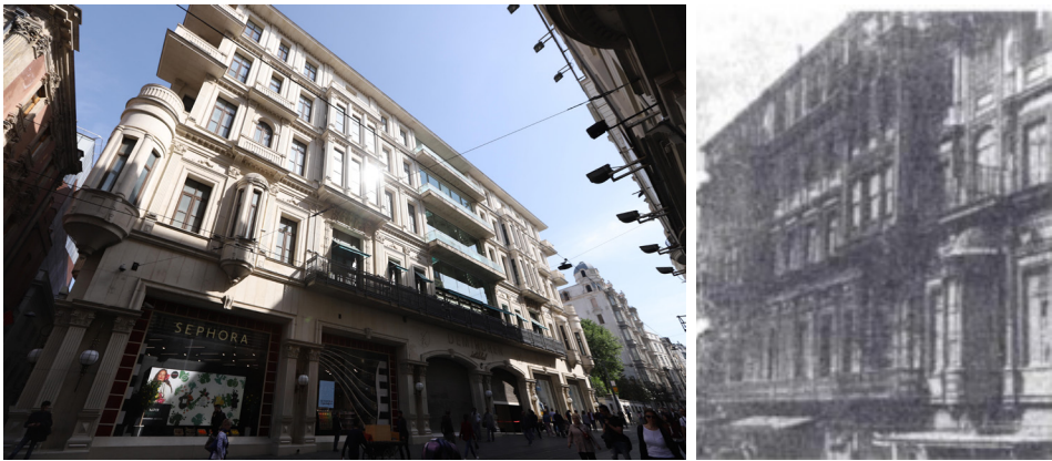
Figura 1. Antic apartament Deveaux (esquerra). Centre Comercial Demirören (dreta). Font de la foto: Autor Figure 1. Left. Former Deveaux Apartment. Right, Demirören Shopping Mall (Photo Source: Author)
