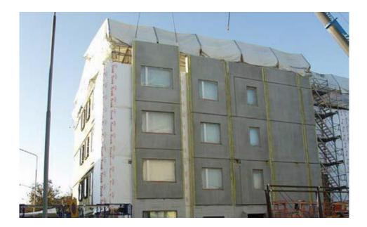
Fig. 10 Protected roof structure with a temporary tube structure
