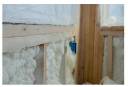
Figure 52 Cavity wall insulation with polyurethane foam <sup>[27]</sup>
