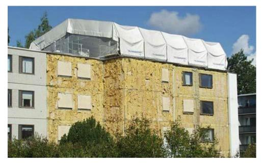
Fig. 6 Demolition of old insulation and outer pane of facade
