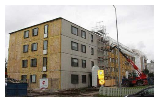
Fig. 5 Demolition of old insulation and outer pane of facade
