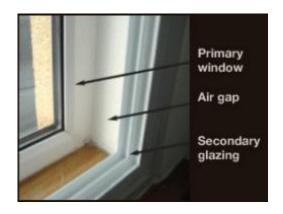
Figure 60 Secondary glazing system [33]
