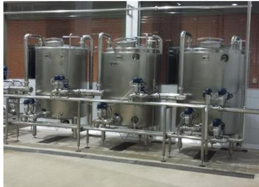
**Figura 7. Sistema de limpieza CIP (Clean in place) (ZUMEX, 2019)**
